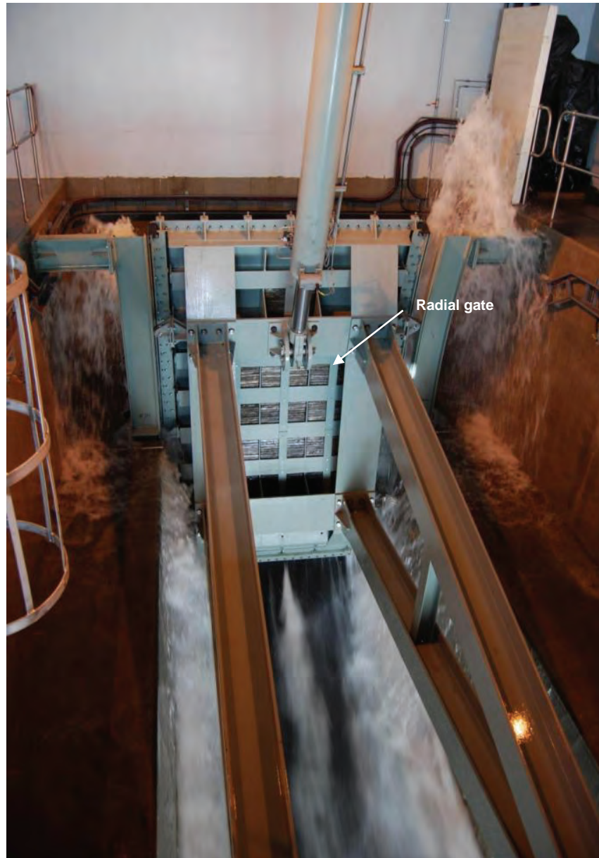
Photo 11: Inside radial gate chamber
