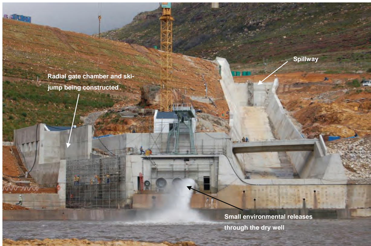
Photo13: Berg River Dam outlet structures during construction phase
