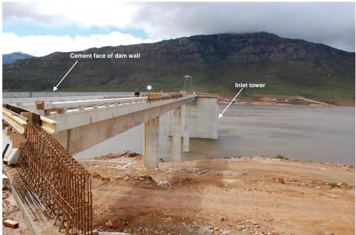
Photo 14: Inlet tower (wet and dry well) and bridge to inlet tower under construction
