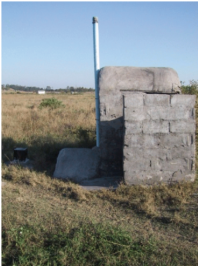
Figure 1: The pit latrine (in use for more than five years), around which monitoring for groundwater contamination took place over a fourteen-month period. The first monitoring hole, just one metre from the pit, can be seen on the left.
