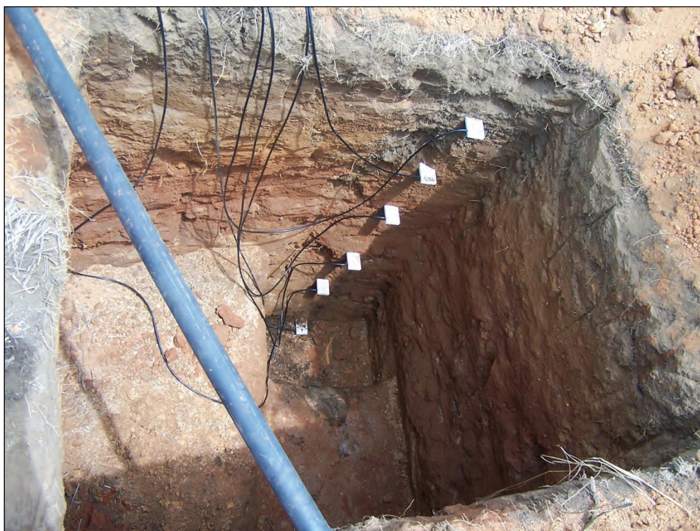
Figure 3.14. Pit excavated to a depth a 2.5 m at the centre of the scintillometer path at Two Streams for the installation of CS616 probes at 0.4 m intervals.
