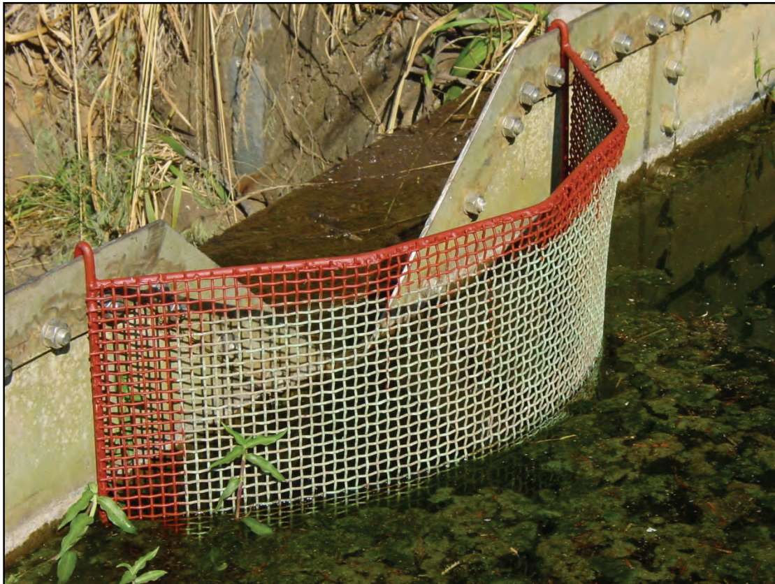
Figure 3.10. A sieve in the main weir at Two Streams kept leaves and branches, which affect the level of the water in the weir, from getting trapped in the V-notch.
