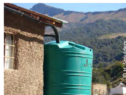
Figure 7.22 U-Round guttering used in Cata Village, Eastern Cape
