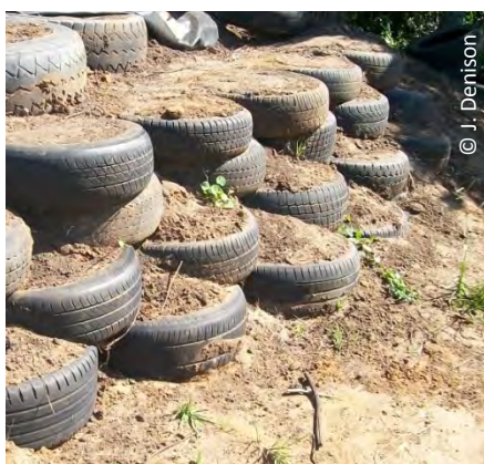
Figure 7.14 A terrace built easily and cost-effectively using old tyres packed with soil.
