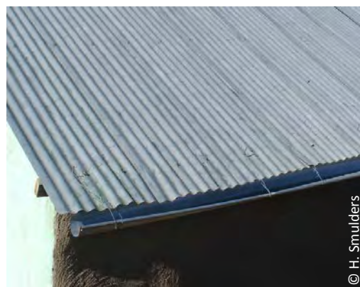
Figure 7.21 Sheet metal gutter fixed to roof sheets with 3mm fencing wire
