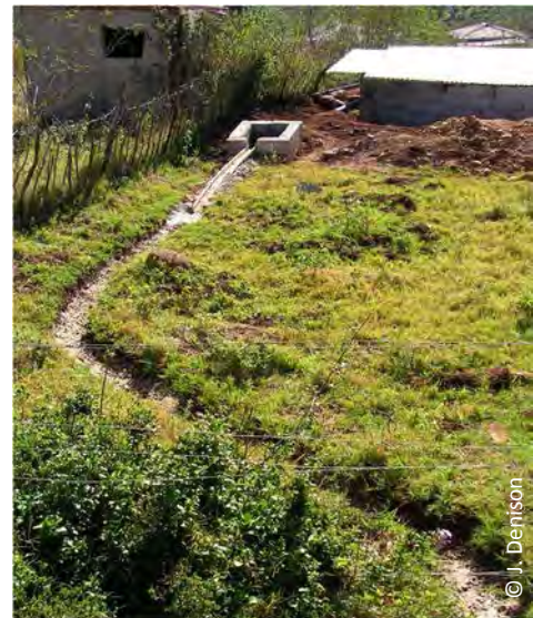
Figure 7.1 Diversion furrow leading to a catchpit
