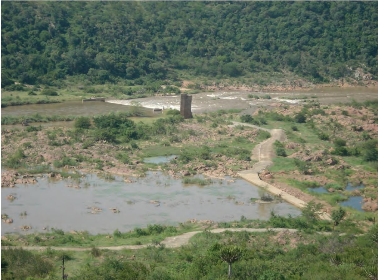
**Photo 7: The gauging weir monitoring flows between South Africa and Mozambique at Ressano Garcia. The international agreement is that a minimum of  $2.6 \text{ m}^3/\text{s}$  should flow over the weir**
