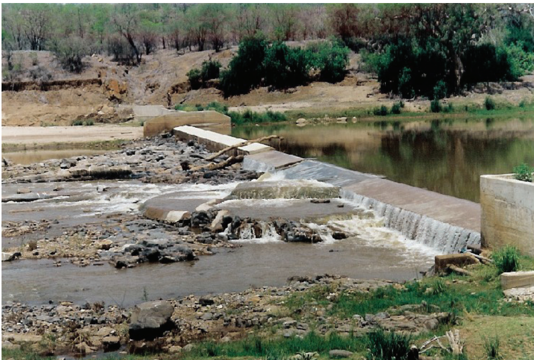
Figure 10-19 Pre-barrage on Olifants River (Bok et al. , 2007)
