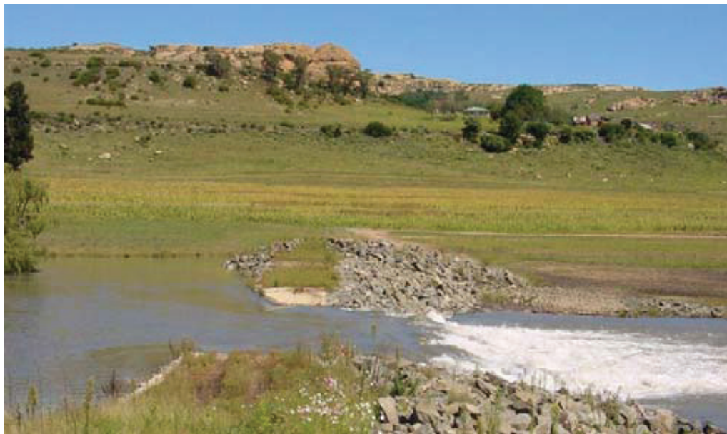
Figure 10-17 Rockfill weir with clay core (after VelaVKE, 2008)
