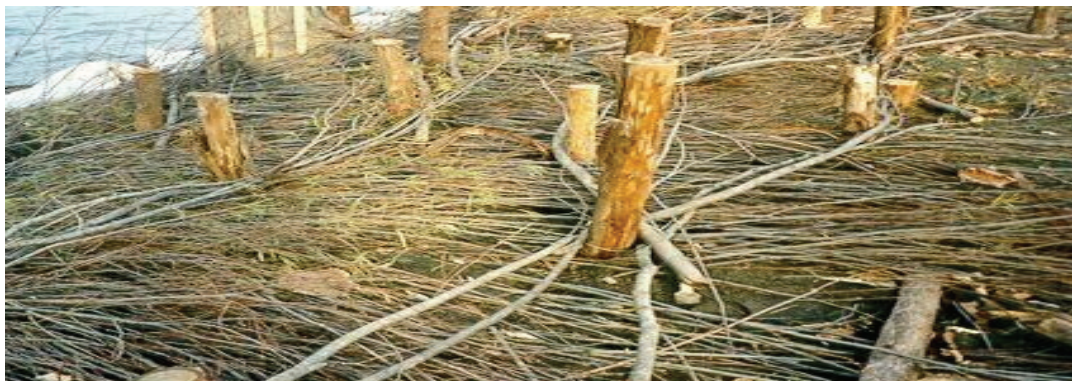
Figure 10-1 Photograph of pegged brush mattress (African Gabions, 2004, in Sieben et al. , 2007)
