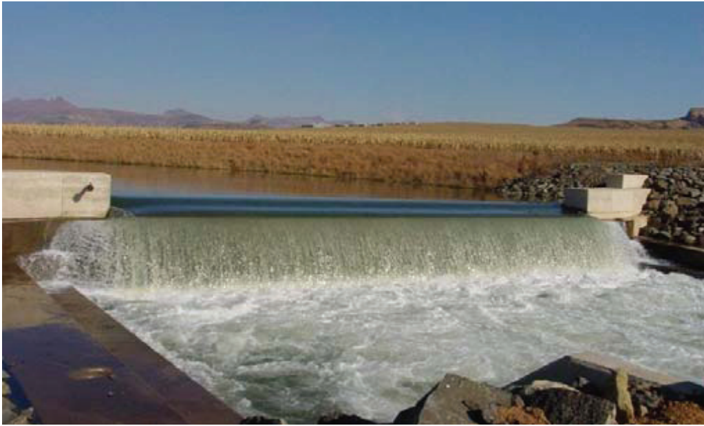
Figure 10-16 Concrete weir on the Ash River to dissipate energy within the channel (VelaVKE, 2008)
