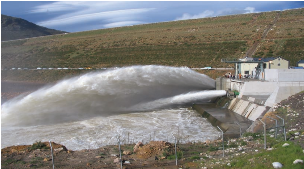
Environmental flows being released from the Berg River Dam
