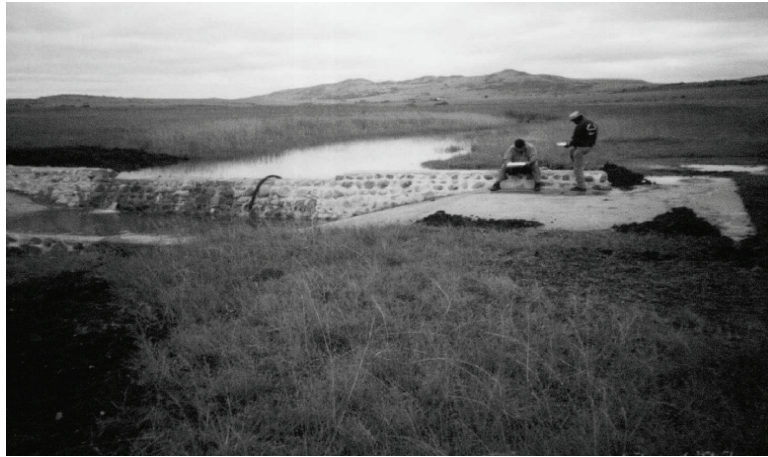
Figure 10-11 Rock masonry weir in a wetland environment (Russell, 2007)
