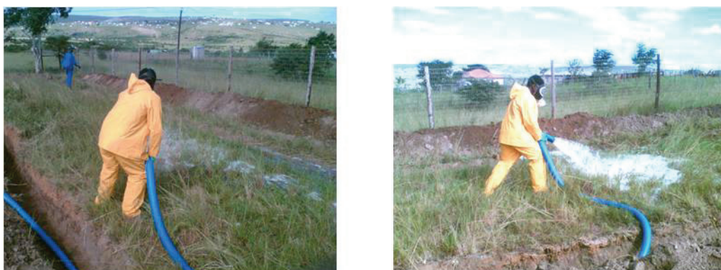
Figure 4:2: Microenterprise employee emptying excess liquid from pits
