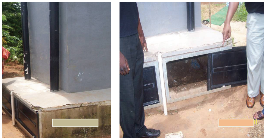
Figure 8: Opening UD vault for maintenance
