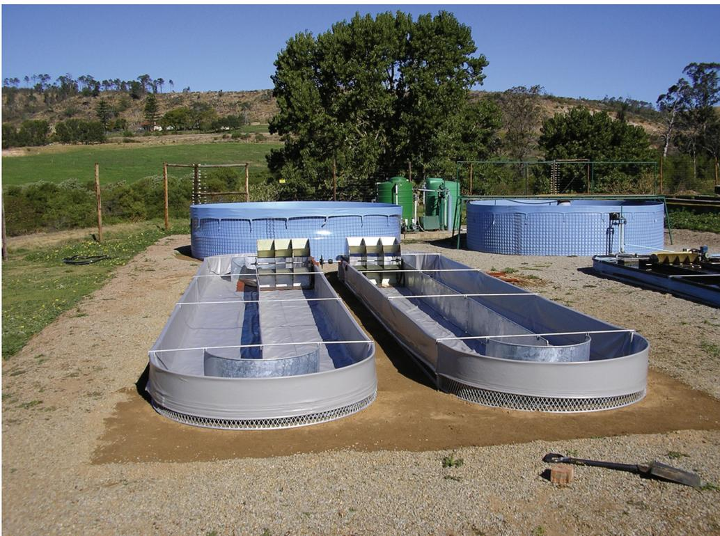
**Figure 3.3:** Installation of High Rate Algal Ponds as components of the new ASPAM pilot plant
