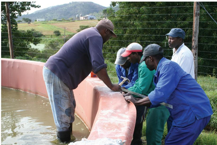
**Figure 3.11:** Fitting of the liner
