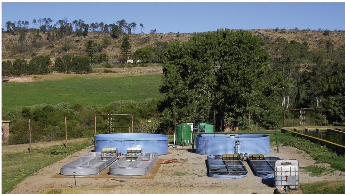
**Figure 3.9:** The retrofitted saline IAPS (right) and the newly constructed ASPAM (left) pilot plants located at the EBRU campus, Rhodes University, Grahamstown
