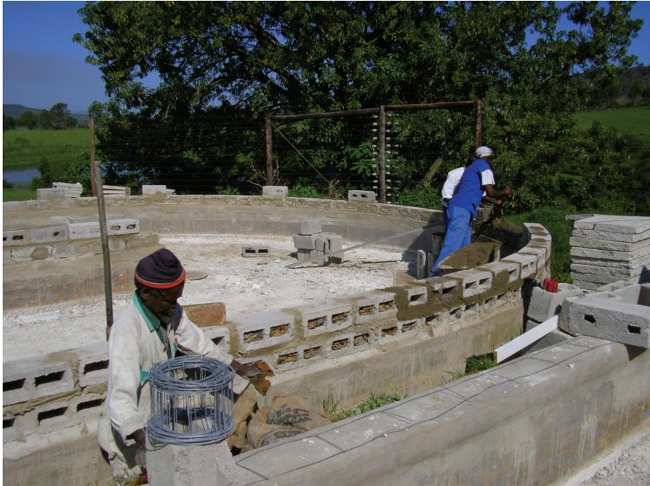
**Figure 3.10:** The walls of the high rate algal ponds were raised with breeze blocks and then plastered
