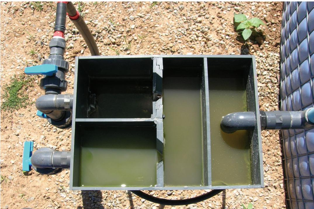
**Figure 3.8:** Splitter box for controlling flow to the high rate algal ponds
