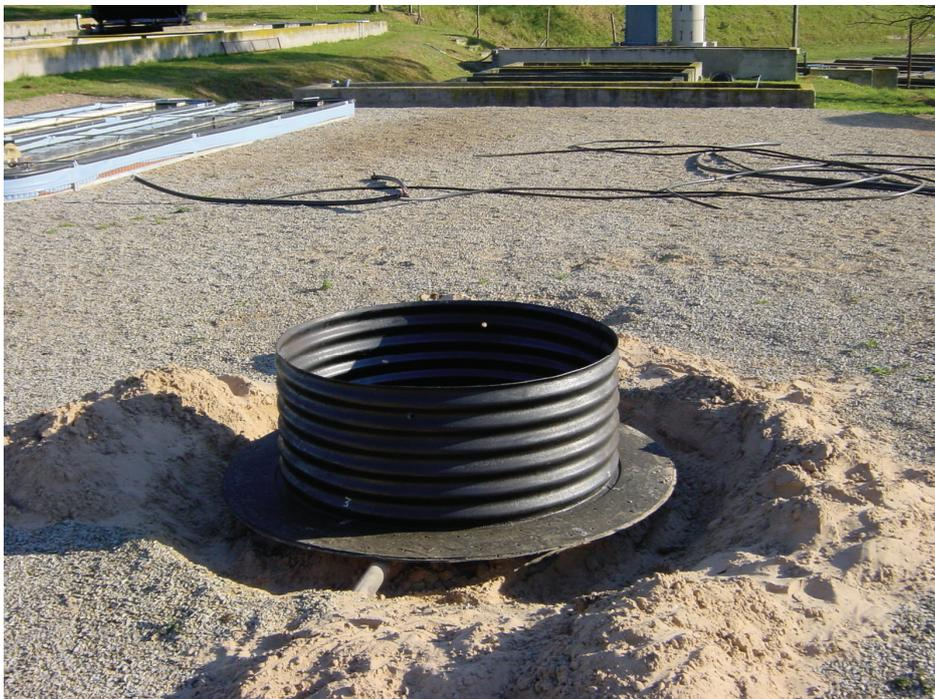
**Figure 3.5:** Installation of the Fermentation Pit component of the Facultative Pond. This is shown prior to the installation of the outer pond works.
