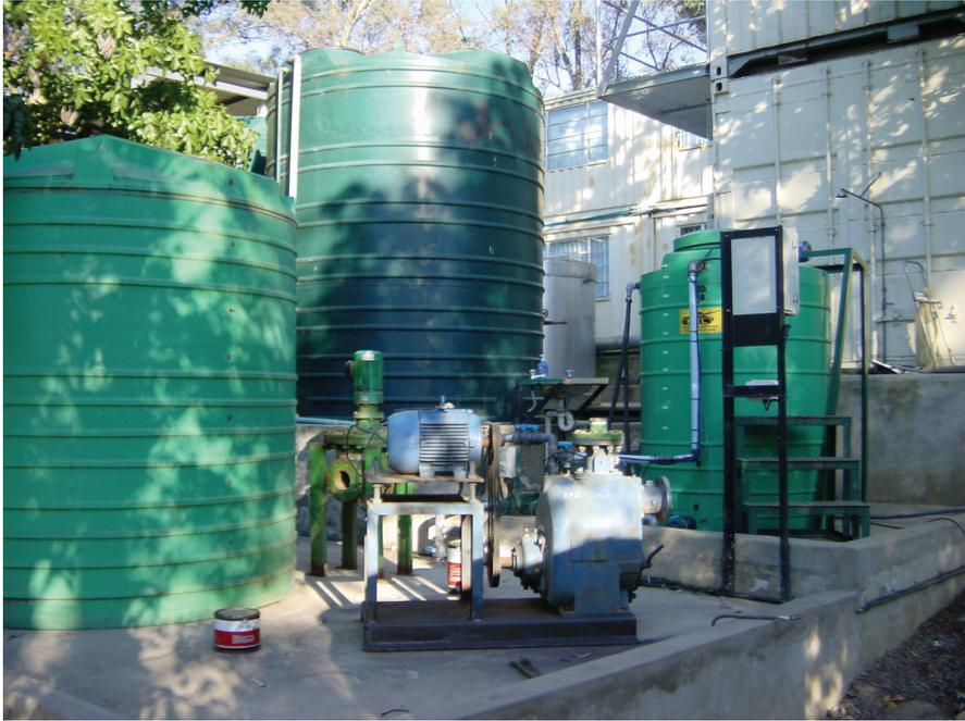
**Figure 3.4:** Make-up and storage tanks for synthetic acid mine drainage wastewater formulation. The influent sewage was macerated in the unit shown in the foreground before feeding to the plant.
