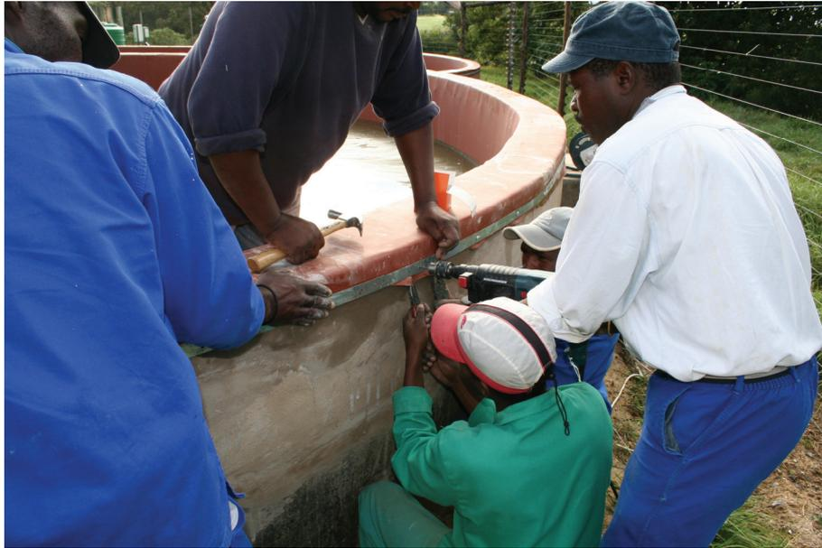
**Figure 3.12:** Securing of the liner
