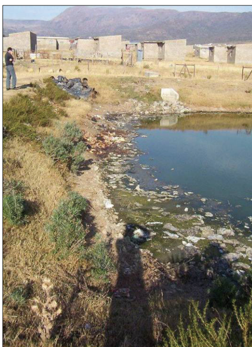
Figure A.16: Old Mt Ayliff Oxidation Ponds
