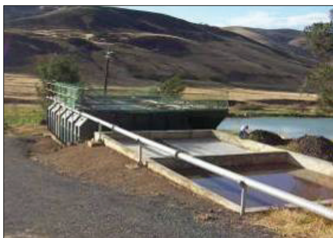
Figure A.19: Package plant activated sludge system at Rietvlei with two piles of sludge visible on the right of the sludge drying beds in the foreground.
