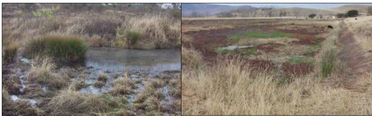
Figure A.18: Clydesdale Oxidation Ponds, showing empty ponds and sewage contaminating a local stream.
