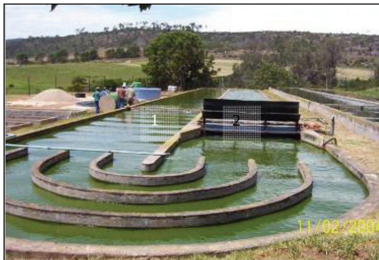
Figure 8.7: View of an High Rate Algal Pond at the Environmental Biotechnology Research Unit field station showing the paddle wheel (1) and motor (2).
