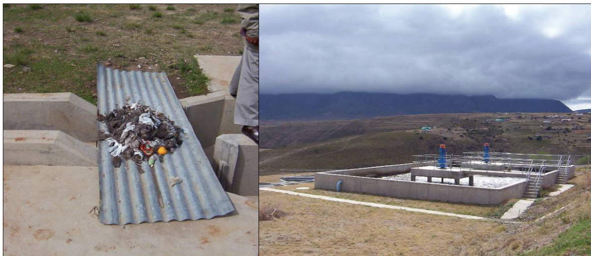
Figure A.17: The new activated sludge system in Mt Ayliff.
