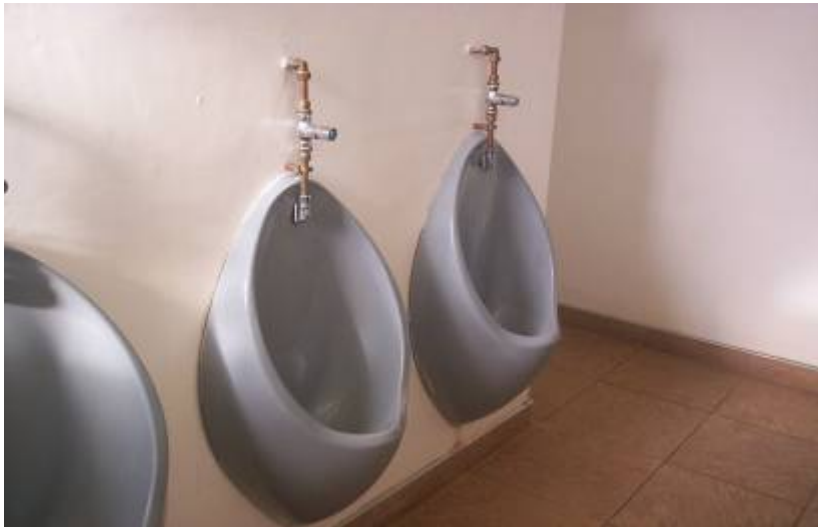
Figure 3.5: Waterless urinals converted to push button flush, Hilton College
