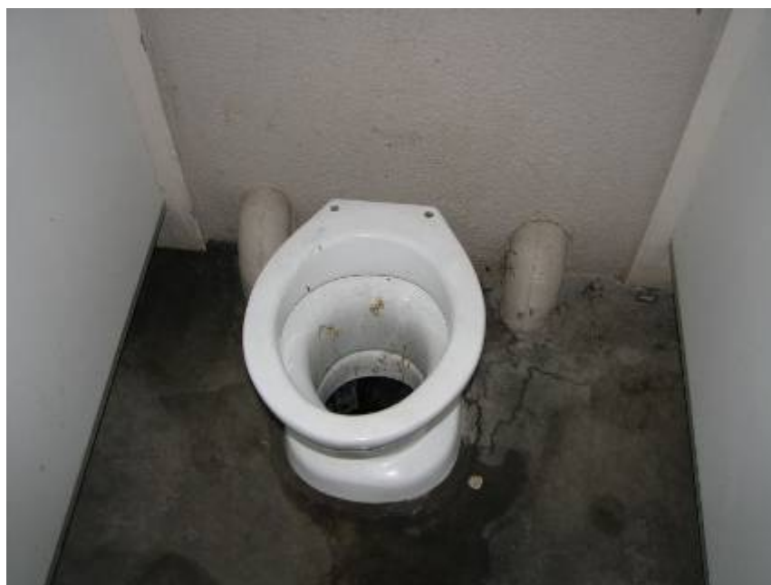
Figure 3.10: A poorly maintained Enviroloo at Signal Hill
