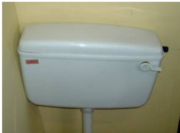
Figure 16: 9 litre single flush cistern
