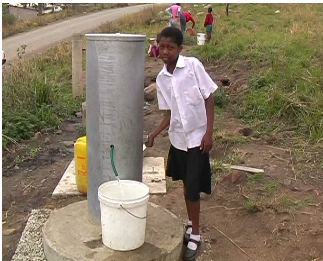
Figure 2.15: The Thelamanzi water efficient public standpipe (manually operated)
