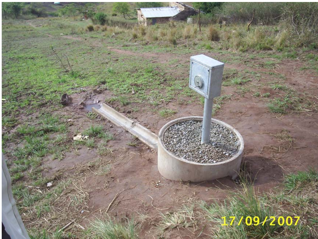
Figure 2.14: The Widget water efficient public standpipe (manually operated)
