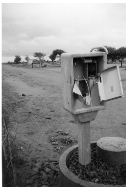
Figure 2.16: Without public buy in, water efficient public standpipes are vulnerable to vandalism
