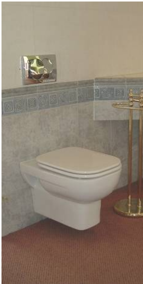
Figure 10: A locally supplied toilet with an imported dual flush mechanism
