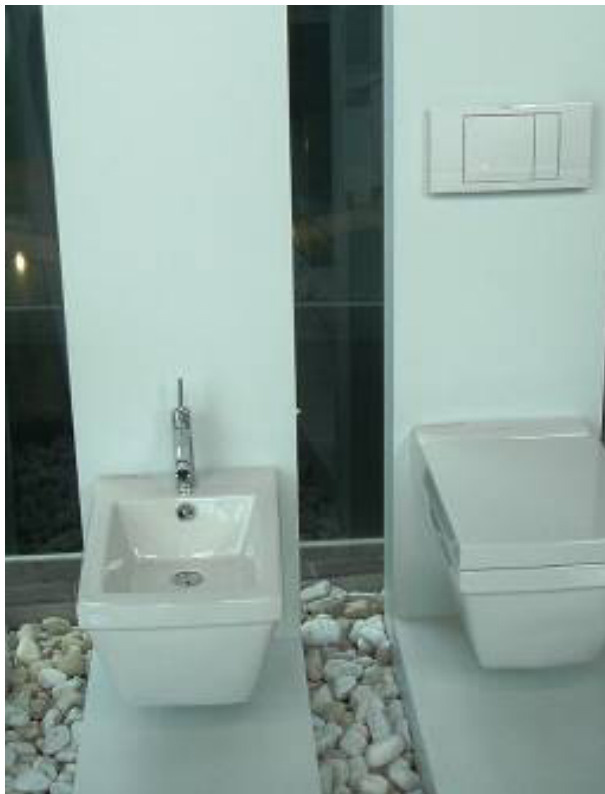
Figure 19: Concealed cistern dual flush 6/3 litre unit and bidet
