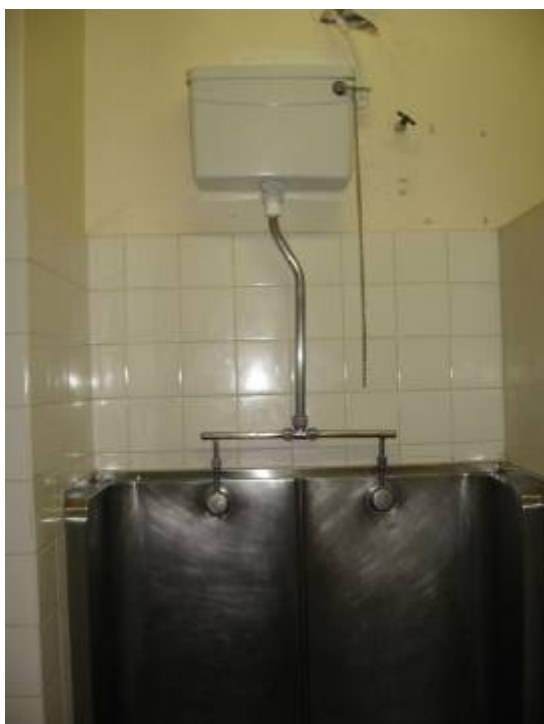
Figure 3.3: An automatic flushing urinal retrofitted to be demand flush
