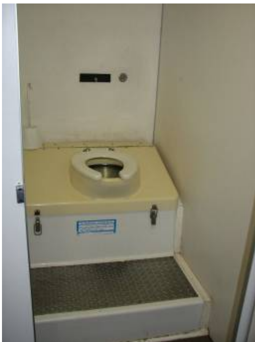
Figure 3.7: A typical container toilet (left) and waterless urinal (right) found at the tourist ablution facilities on Table Mountain
