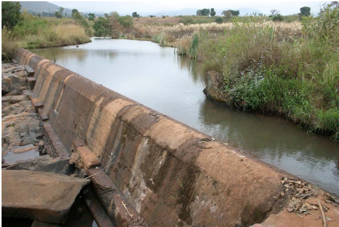
FIGURE 2.6: The concrete weir on the Dzindi River that diverts water to the Dzindi Irrigation Scheme
