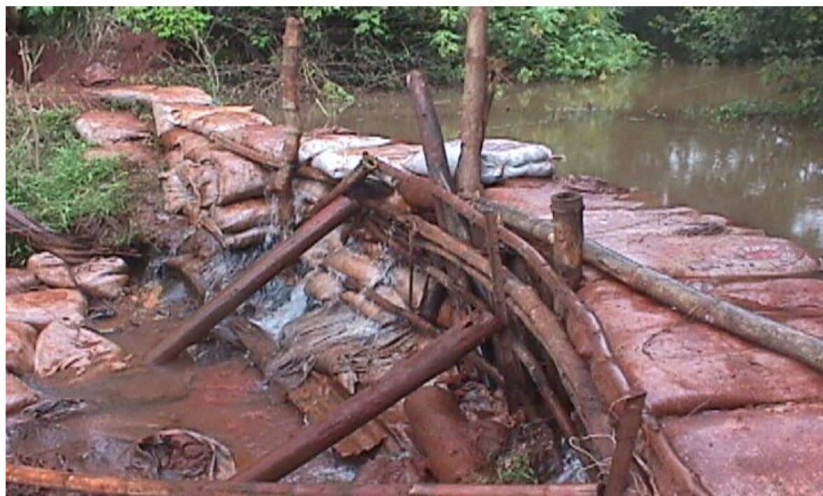
FIGURE 6.3: The weir made of sandbags and wooden poles by a private farmer to extract water from the Dzindi River
