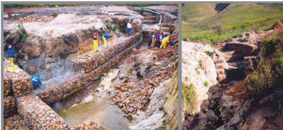
Figure 7: Gabion complex A1-4, at left under construction, at right after completion (2001). It was very stable and well vegetated by 2005, and was slightly damaged in the 2006 flood.
