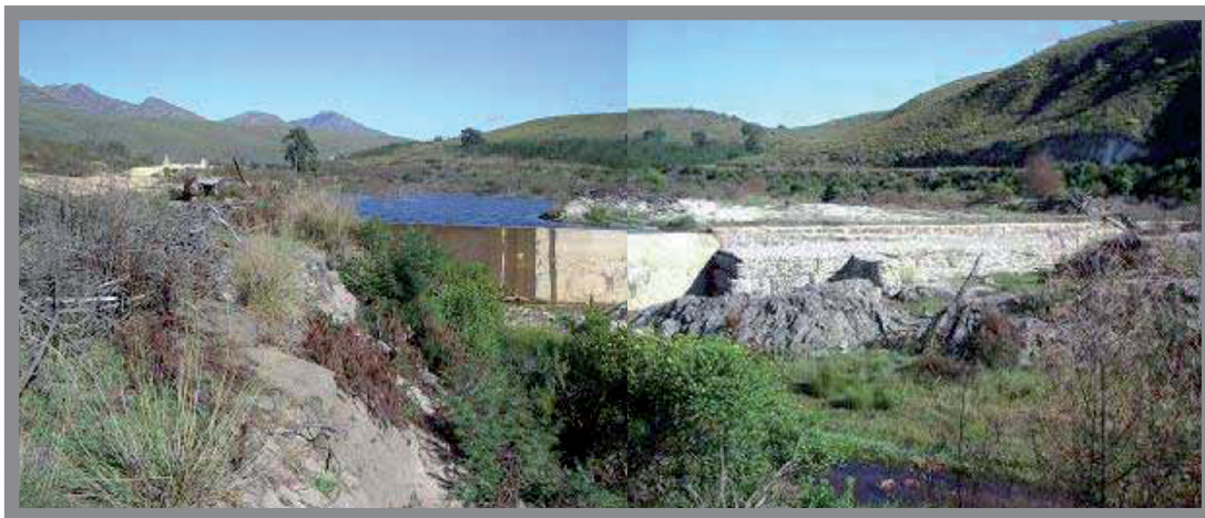
Figure 10: Weir B3 of concrete and rock gabion in the key point at Companjesdrift, below the confluence with the Eerstedrif River (2004)
