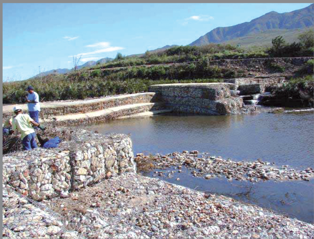
Figure 11: Top: Gabion C at Hudsonvale in 2002. Bottom: Gabion being mended after the 2006 flood. The structure has two main sections with a central support wall. The structure has been stable and survives cattle using it as a walkway to cross the river.
