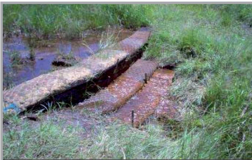
Figure 6.24: Fibre bags used to deactivate gully head erosion. Note the very small step height and downstream impact protection.
