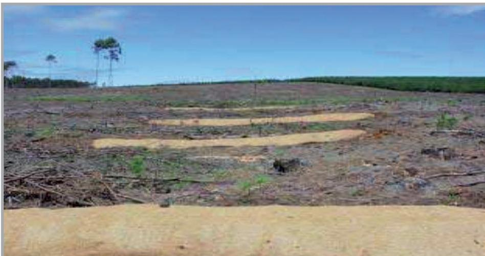
Figure 6.12: Fibre mats covering compacted soil berms in a seepage wetland that previously had been drained
