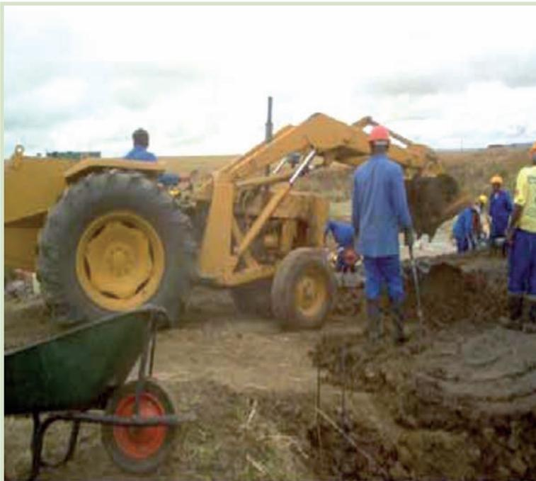
Figure 26.3: Where relatively large earthwork is required, a front end loader will make hand labour more efficient
