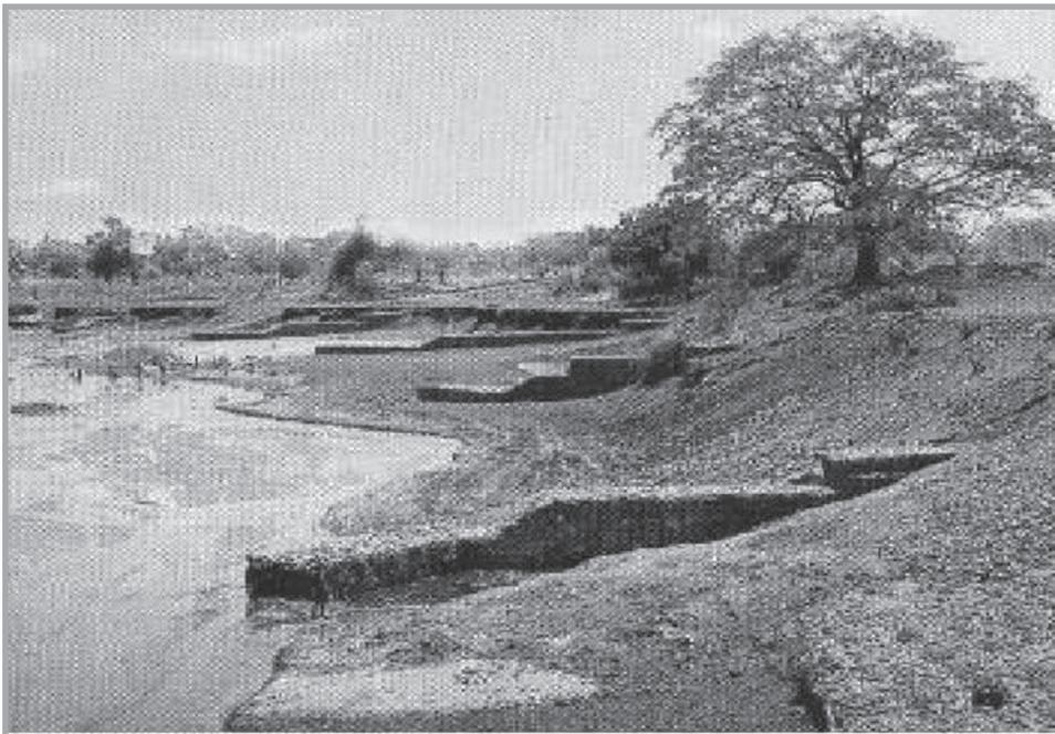
Figure 7.5: A system of gabion river groynes protecting a stream bank
