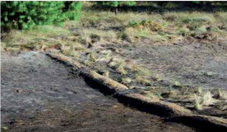
Figure 6.19: Fibre bags placed in sloped area of gully at the London rehabilitation project in Mpumalanga
