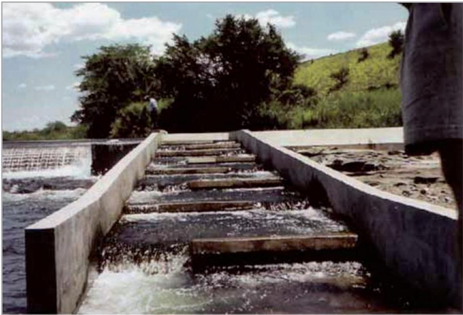
Figure 12.2: Notched weir fishway – Komatipoort
