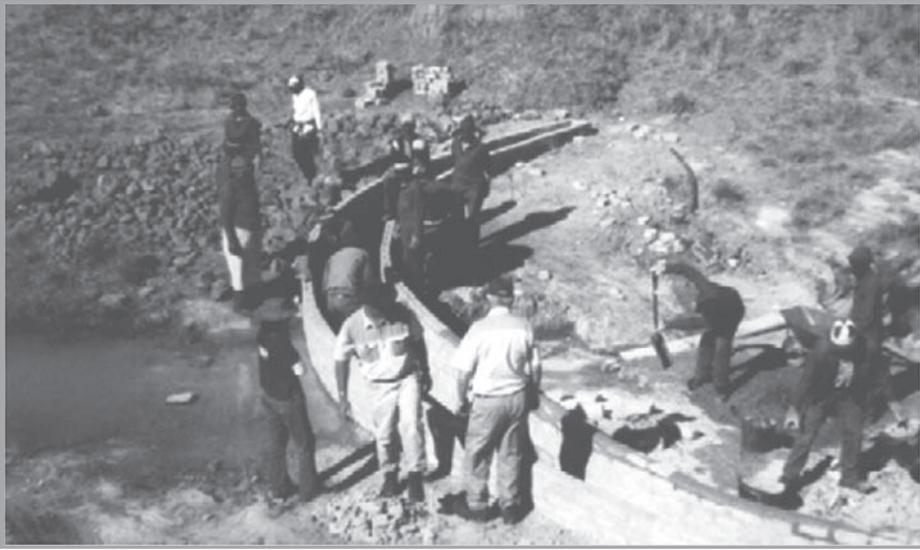
**Figure A 3.2: Building an arch weir. Double walls of concrete bricks with concrete fill in-between. Planned for raising once the sediment has reached the spillway level**
