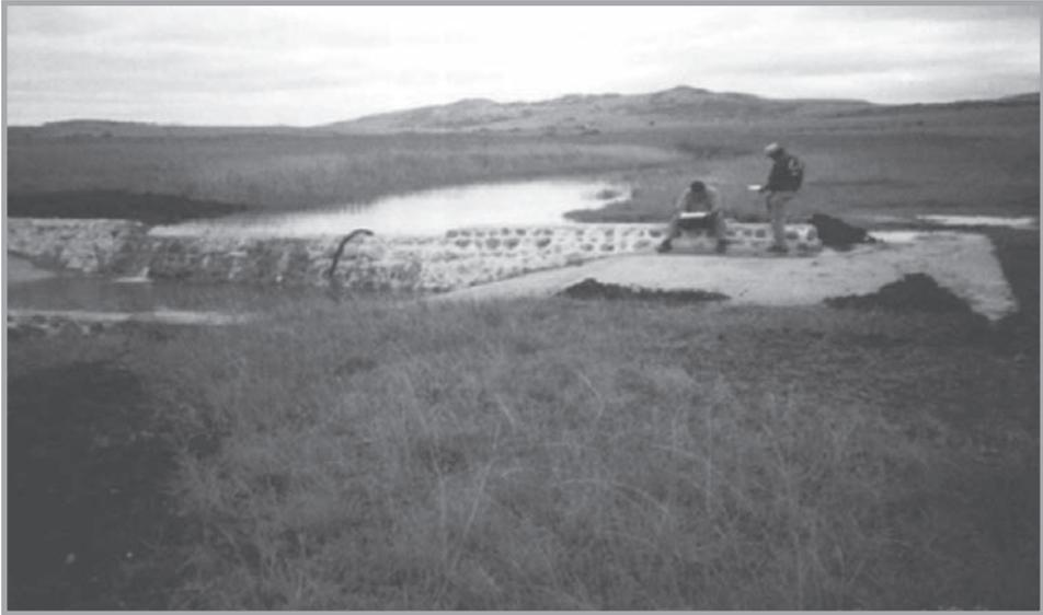
**Figure 28.5: Rock masonry weir**
