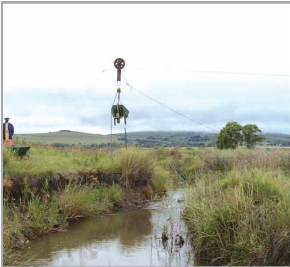
**Figure 29.1:** An innovative and effective method of transferring materials across a wetland using a cableway with a wheelbarrow suspended from it.
