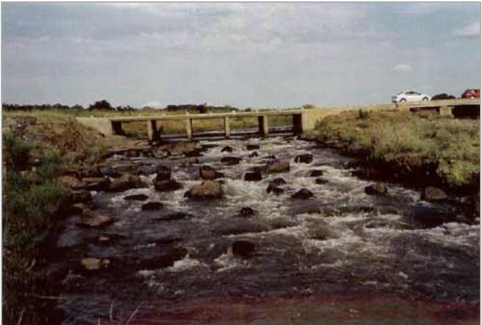
Figure 12.41: Bypass Rockramp fishway – KNP
