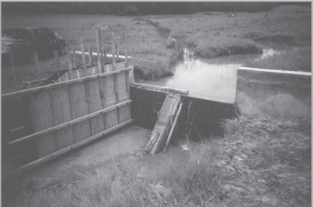
Figure A 3.4(b): The wall and buttress complete, the shoulder walls are now being built, as indicated by the position of the shuttering
