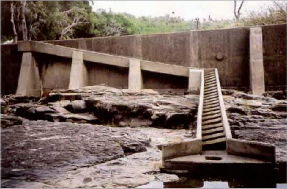
Figure 12.7: Haga-Haga river pool and sloping weir fishway designed for small fish (<120 mm long)
