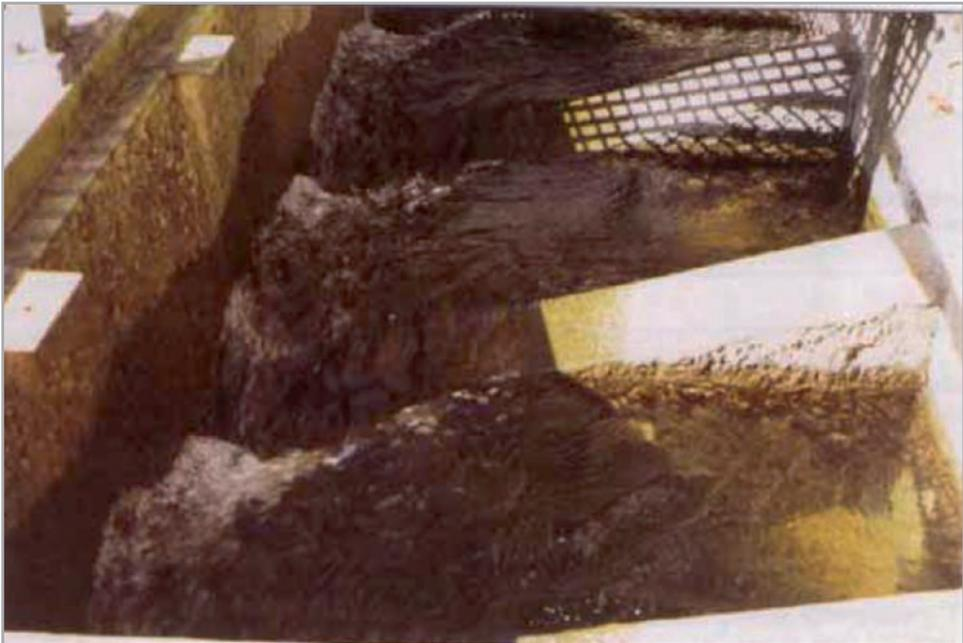
Figure 12.8: Close up of sloping weir of the Nhlabane pool and weir fishway at low flows, looking upstream
