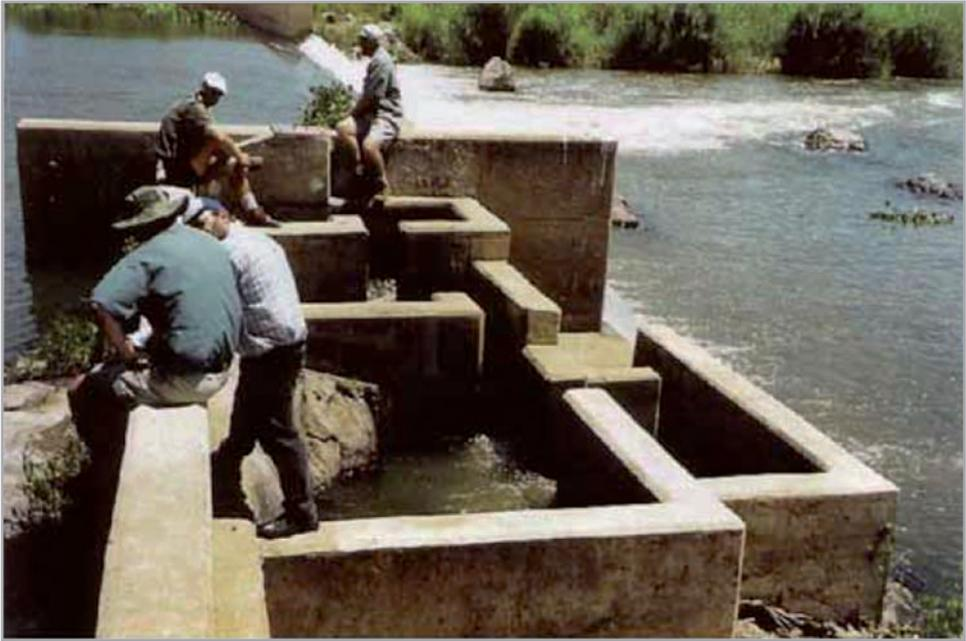
Figure 12.3: Pool and slot fishway – KNP
