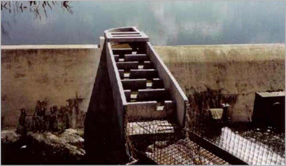
Figure 12.1: Notched weir fishway under construction – Komatipoort
