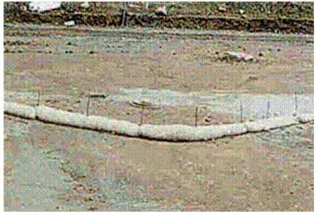
Figure 6.17: Fibre rolls pegged in position on bare soil ([www.beltonindustries.com](http://www.beltonindustries.com))
