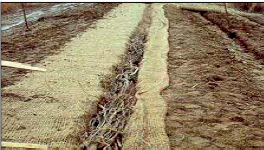
Figure 6.7: Installing live vegetative bundles on a slope with coir netting (African Gabions, 2004).
