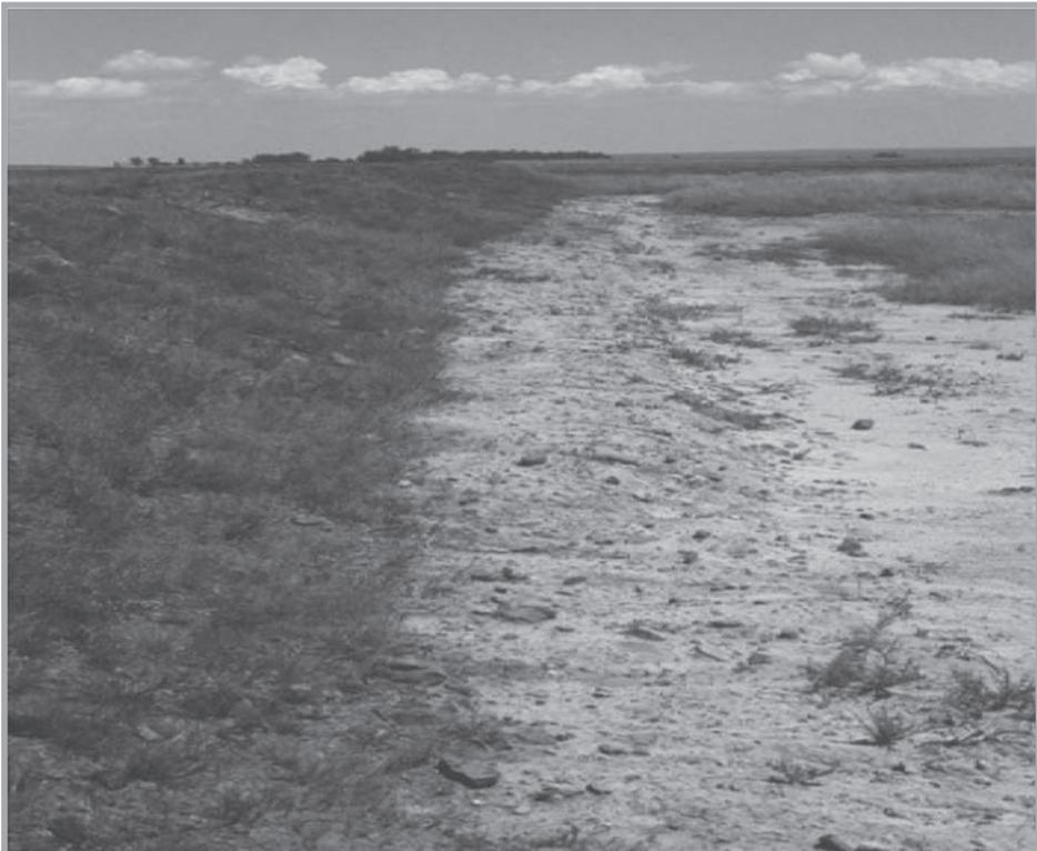
**Figure 28.4:** Effect of a gravel blanket on an earthen berm in an arid climate. The upper half is covered in rip-rap, is colonized by vegetation and is stable. Whereas the lower half is not covered with rip-rap. The soil is bare and is being eroded and washed away.
