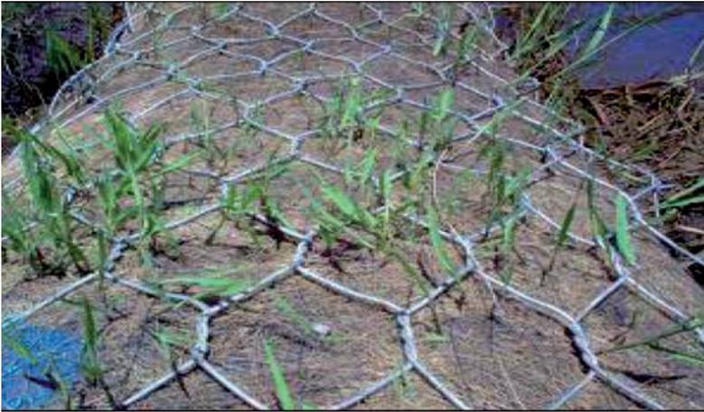
Figure 6.18: Fibre bag with wire sheath. Vegetation can be seen emerging from the top soil in the bag.
