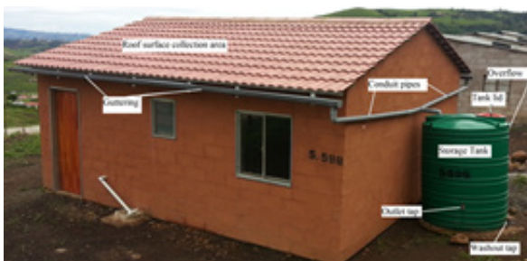
Figure 1 – A typical rooftop rainwater harvesting system.
