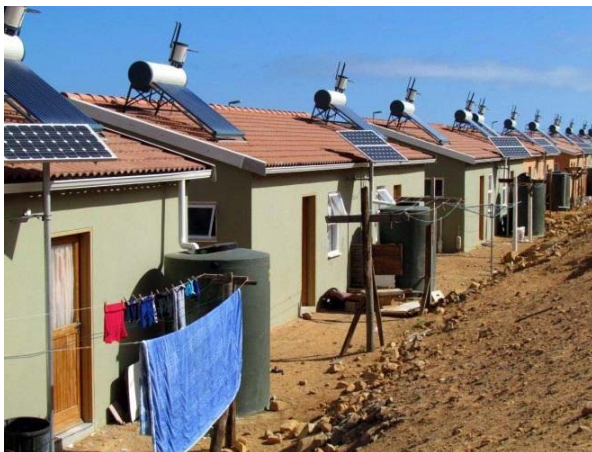
Domestic rainwater harvesting systems in Kleinmond, Western Cape.
