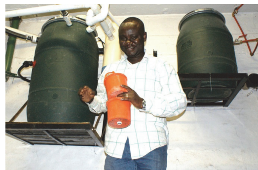
Ola Olanrewaju of Wits University working on the pilot dual grey- and drinking water reticulation system.
