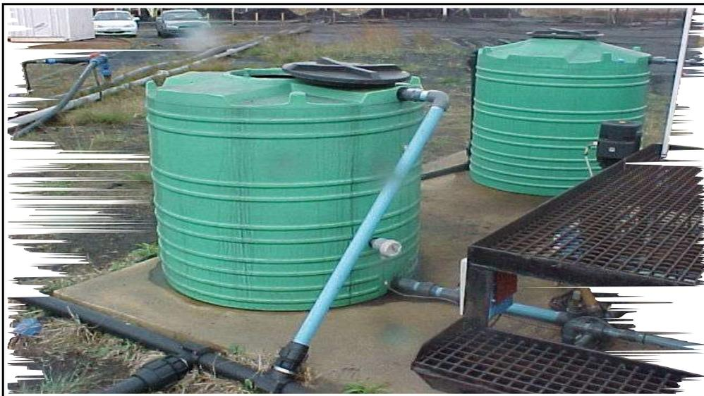
**Photogram 2: Mine Water Feed Tank**
