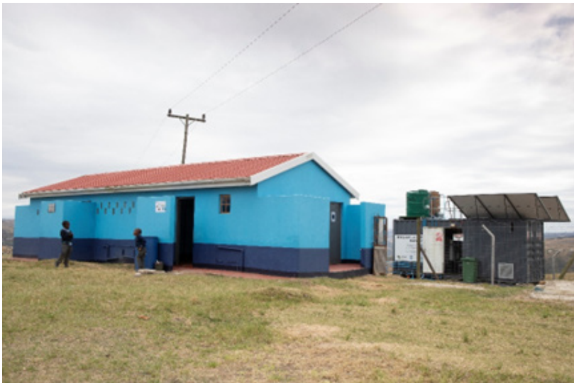
Example of a WESS system at a school. Note the treatment unit to the right.
