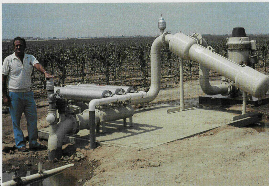
Drip irrigation in a vineyard in California showing the pump and filter system and an irrigated grape plant.
