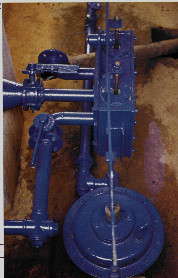
The Turner gate, a locally designed automatic compensating demand sluice maintaining constant canal water head in Gamtoos GWS.
