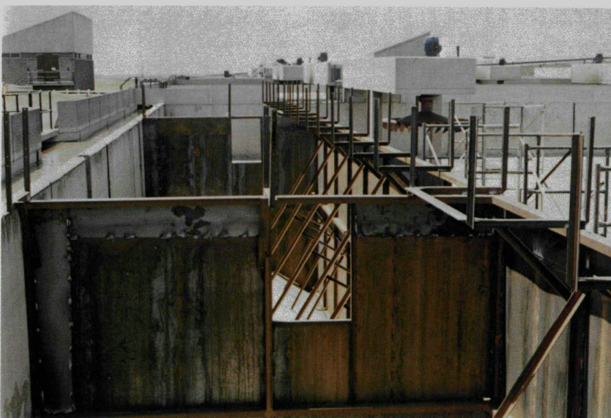
The three-compartment selector under construction.
