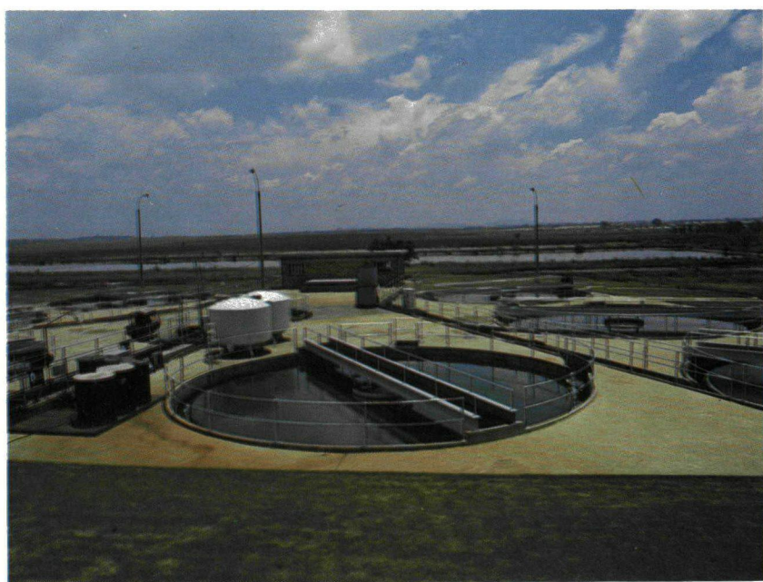
Three humus tanks and chemical dosage system used in the preliminary phosphate removal studies.
