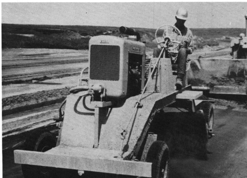
A typical soil-cement placing train ploughing a soil-cement slope protection on an embankment dam in the USA. Similar equipment would be used in constructing the soil-cement dam envisaged by Dr JA Robertson.
