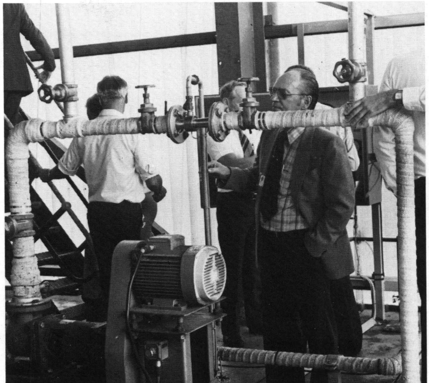
Mr FS Vivier, Department of Health and Welfare, closely inspecting the Vitox oxygen injection venturi of the autothermal aerobic process.
