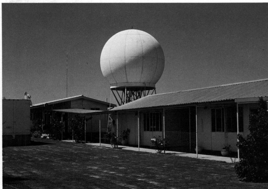
Part of the Bethlehem research station. The huge white "ball" is the radome which houses the project radar. The radar is used to record the three dimensional characteristics and behaviour of clouds in the area.
