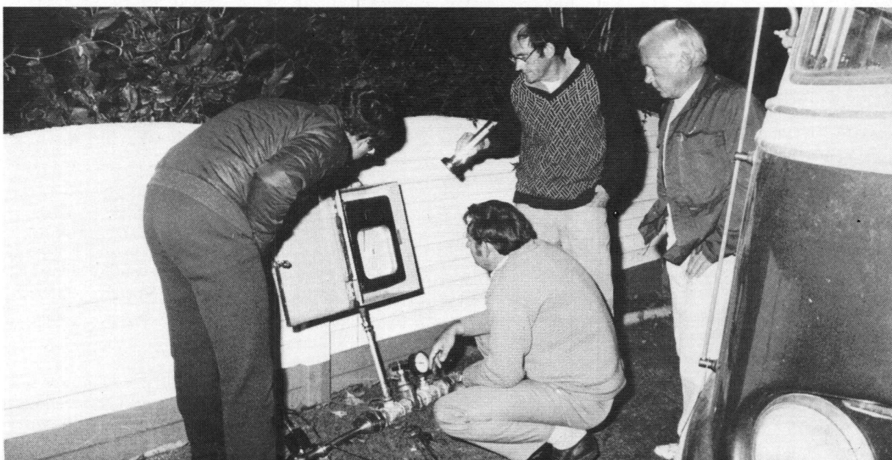
(From left) André Marais, Paul Odendaal, Charles Chapman and Pieter Swanepoel observing the pressure drop test necessary to confirm total isolation of the area.
