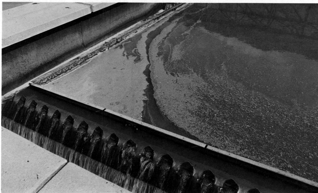
A close-up view of the sedimentation tanks showing the discharge of settled sewage and the removal of floatables prior to the discharge to sea.
