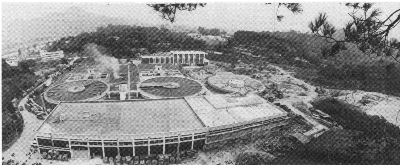
Work in progress for upgrading a water treatment plant at Tuen Mun, one of the seven new towns being developed in Hong Kong.
