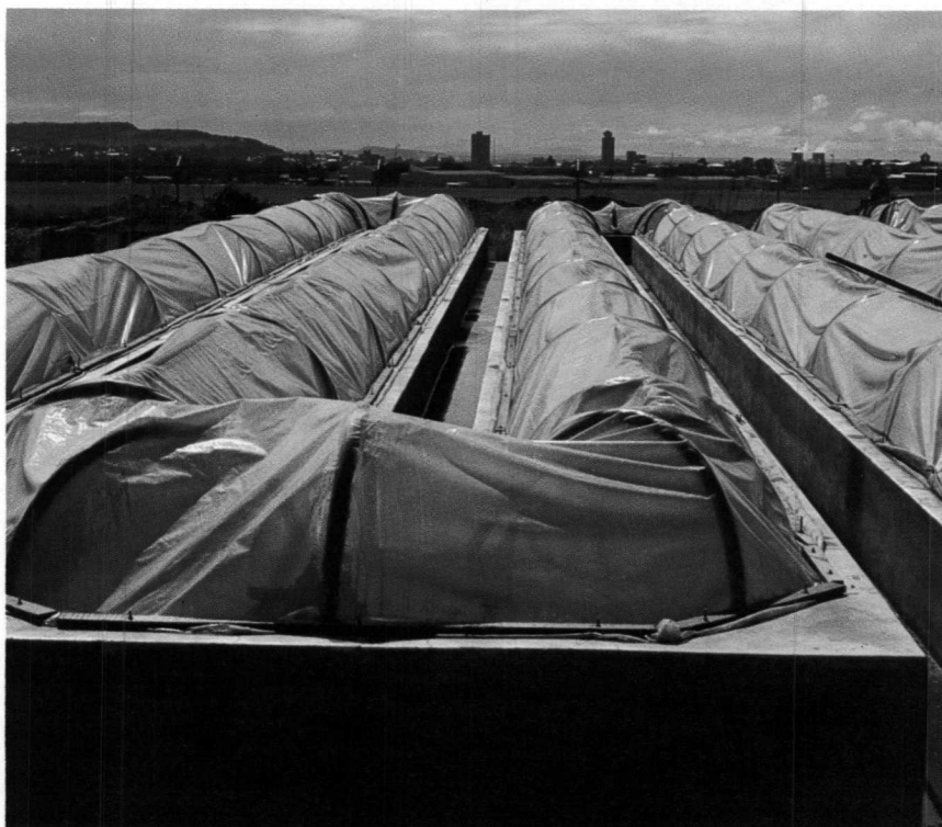
(Opposite page and below) 100 m 3 plastic-covered pilot pond on the University of the Orange Free State's experimental site.
