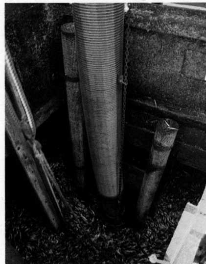
The suction pipe used for offloading an anchovy harvest at the Suid-Oranje factory, St Helena Bay.
