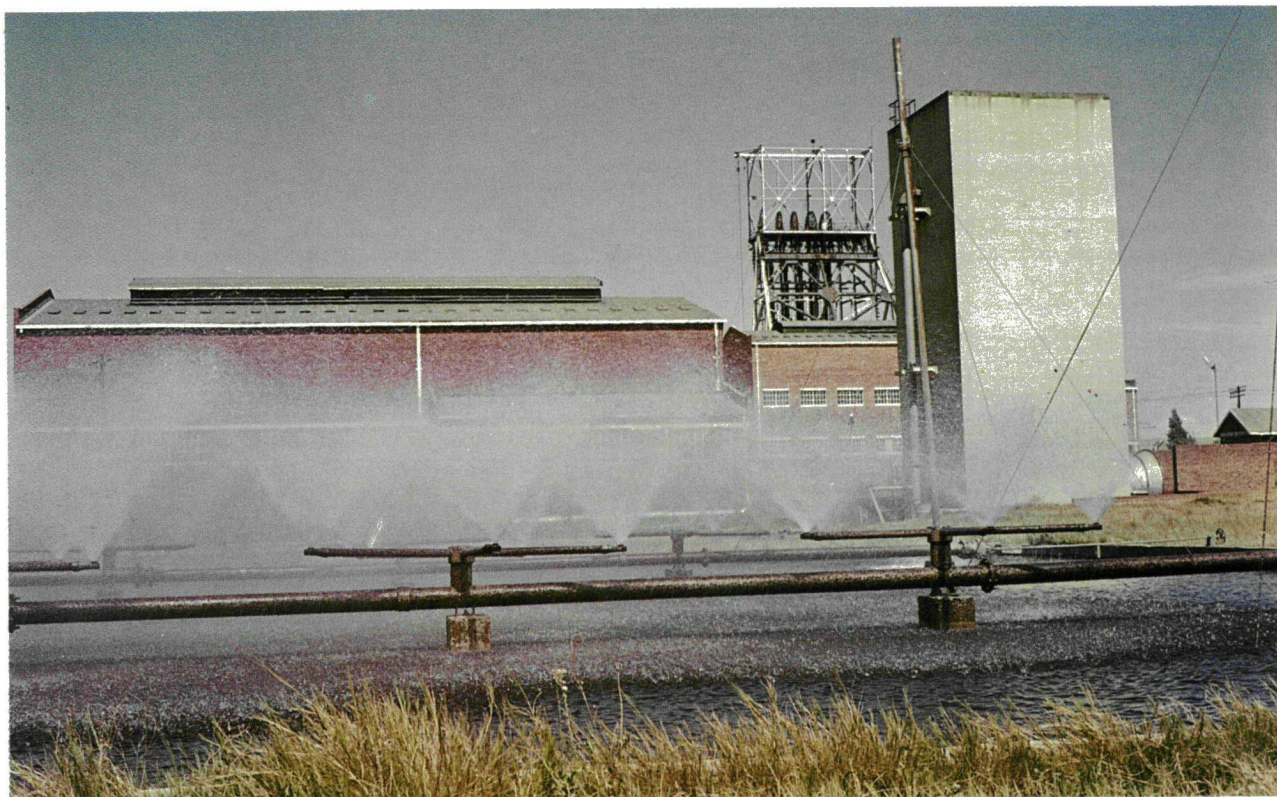
Spray cooling pond for cooling compressed air.
