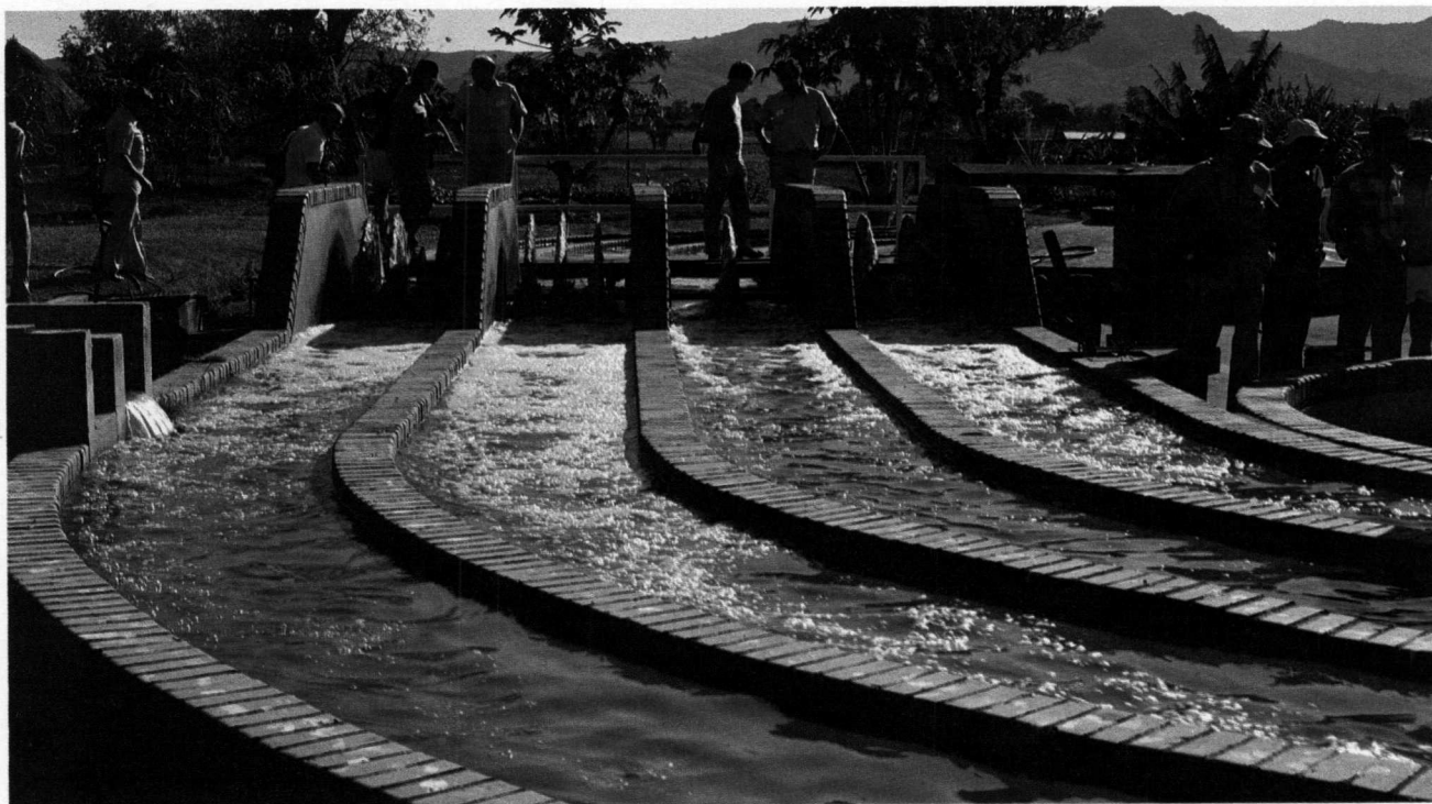
The four-channel activated sludge Orbal system at the Tshlidzini Hospital.
