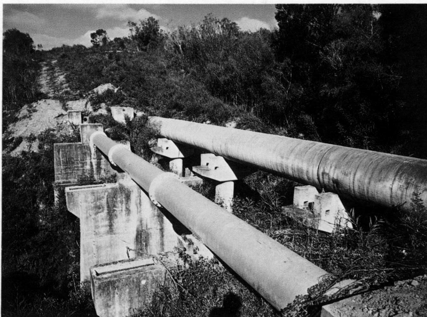
The steel pipeline on the left has recently been reconditioned by cement mortar lining in situ.
