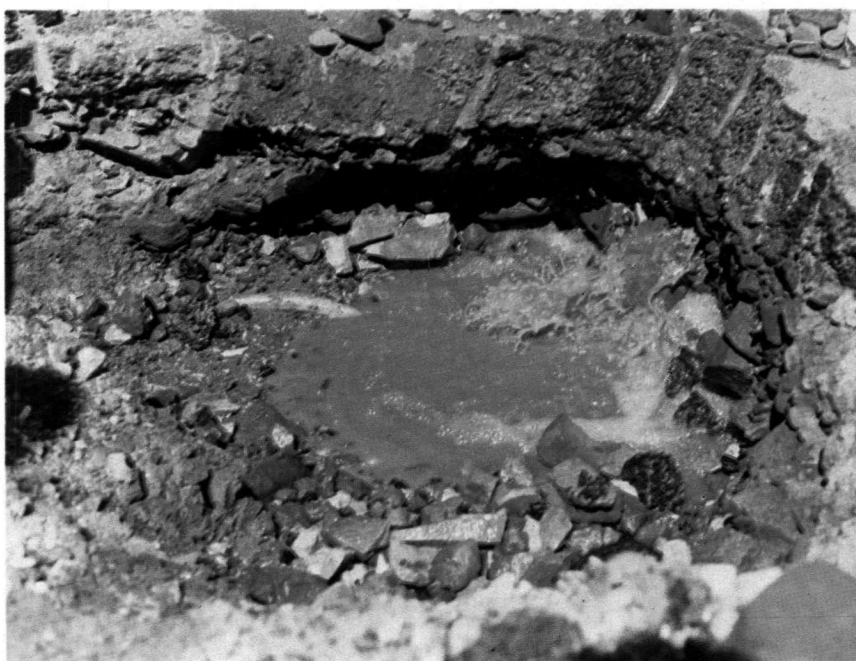
A hidden leak after excavation.
