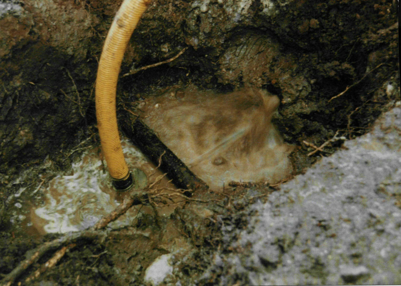
This leak in a small diameter main running underneath a tarmac road surface, was detected with leak detection equipment.
