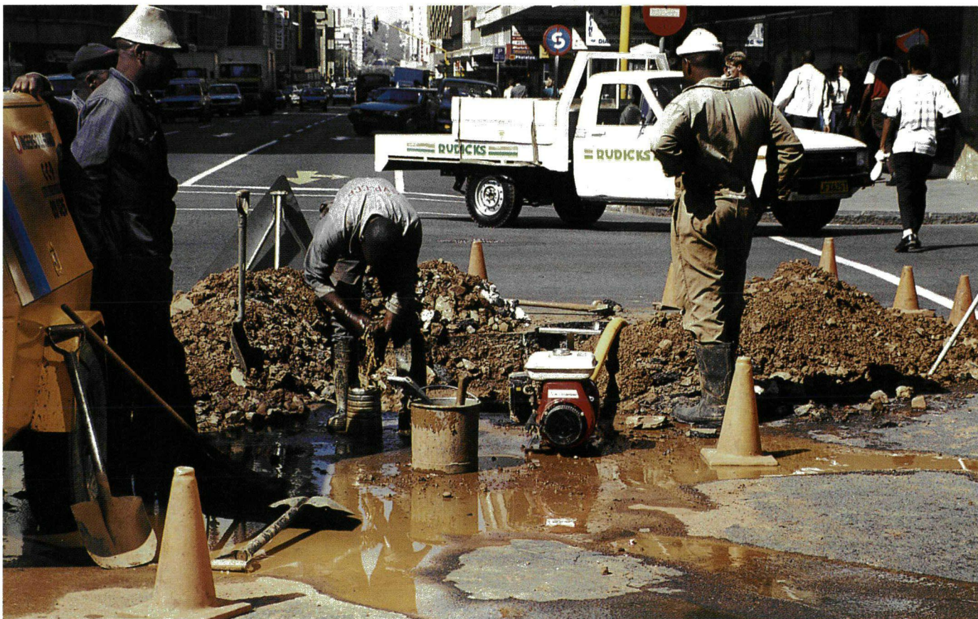
A leak detection team in action.
