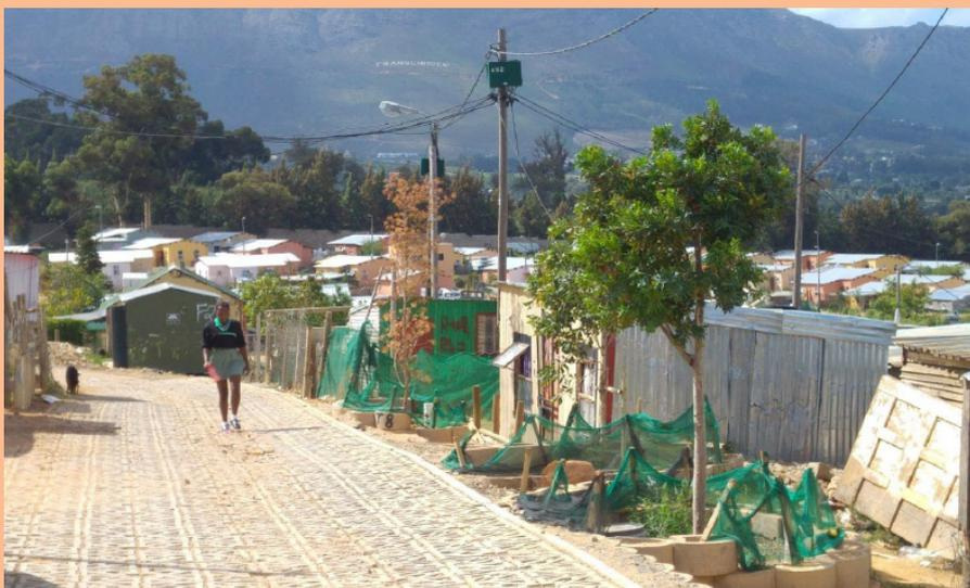
Permeable paving constructed between homes in the informal settlement of Langrug, near Franschhoek, South Africa. Surface hardening leading to poor infiltration, coupled with poor water management systems resulted in wastewater and sewage flowing through the streets. This was addressed with an integrated green and grey infrastructure approach: a combination of permeable pavements, wastewater management systems and insertion of pipelines.
