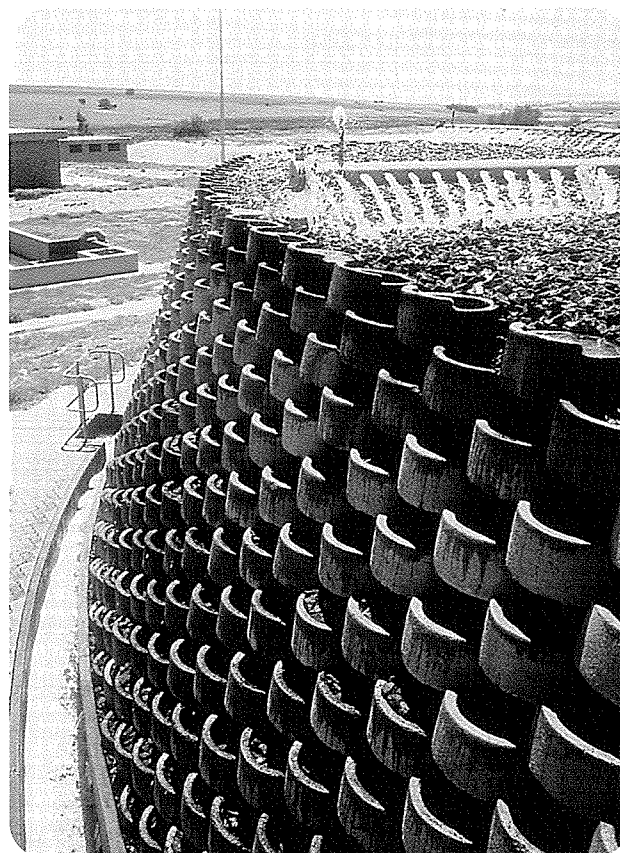
Wastewater distribution across a modern biofilter.
