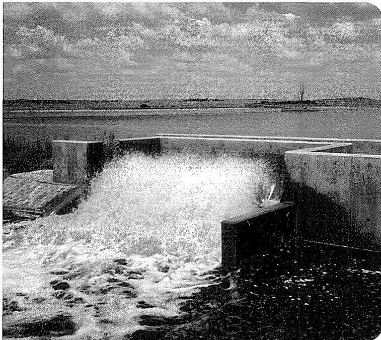
A key factor for the low-tech generation of readily biodegradable organics in the envisaged BNR PETRO concept: Algae-rich recycle provided to the surface of the primary pond (Bloemfontein).
