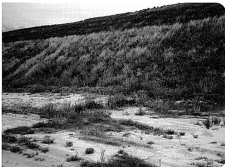
Field plots for the evaluation of different approaches to slime dam rehabilitation.
