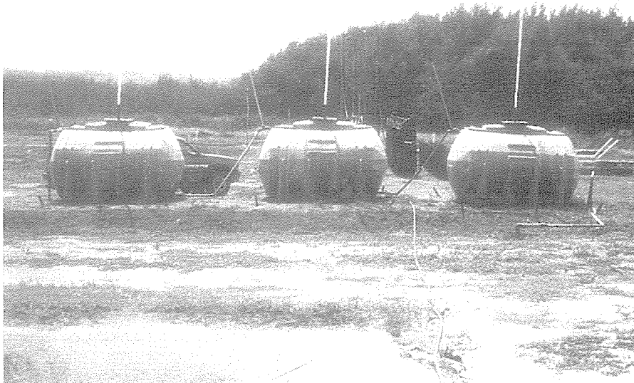
The anaerobic contact bed / anoxic limestone drain (ACB/ALD) train which was used to neutralise acid mine water for use in additional experiments, conducted at Arnot Colliery, to develop integrated passive water treatment systems for mine effluent streams.
