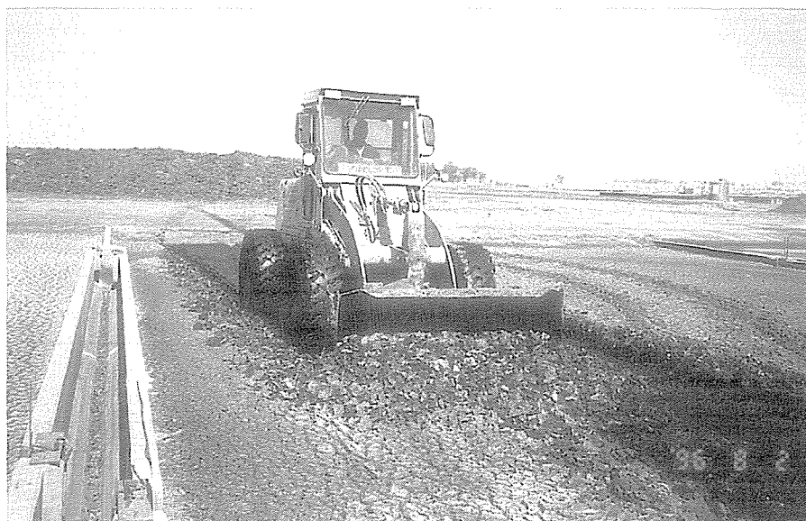
This photograph illustrates the advantages of mechanical removal of sludge. The sludge is removed at higher moisture contents than compared with manual methods and is clearly more efficient than the latter.
