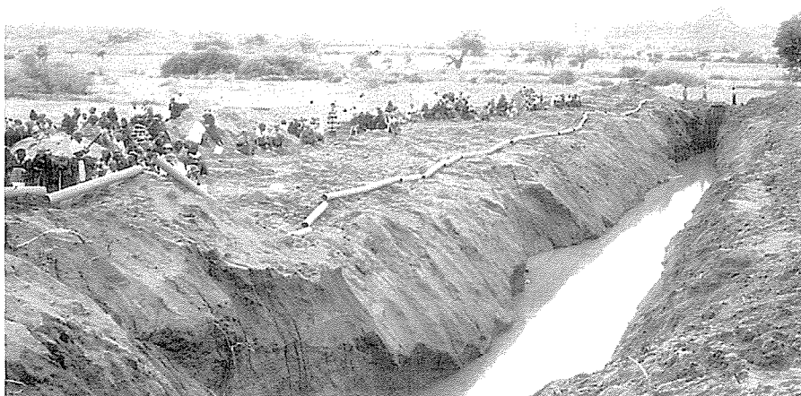
Community-based construction of a shallow infiltration gallery in the Nebo District, Northern Province. The supply from the gallery is in the order of 2,0 l/s in an area where average yields are between 0,5 l/s to 1 l/s. The water is, in addition, free of fluoride, opposed to high fluoride concentrations from conventional boreholes located in the young granite.
