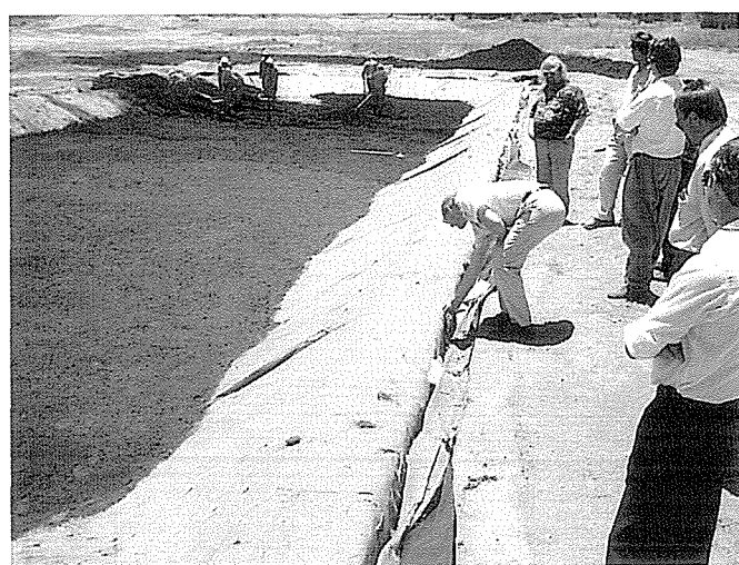
The construction of an integrated passive water treatment system for mine effluent streams.
