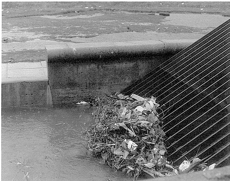
Trash racks for the removal of floating and suspended materials.
