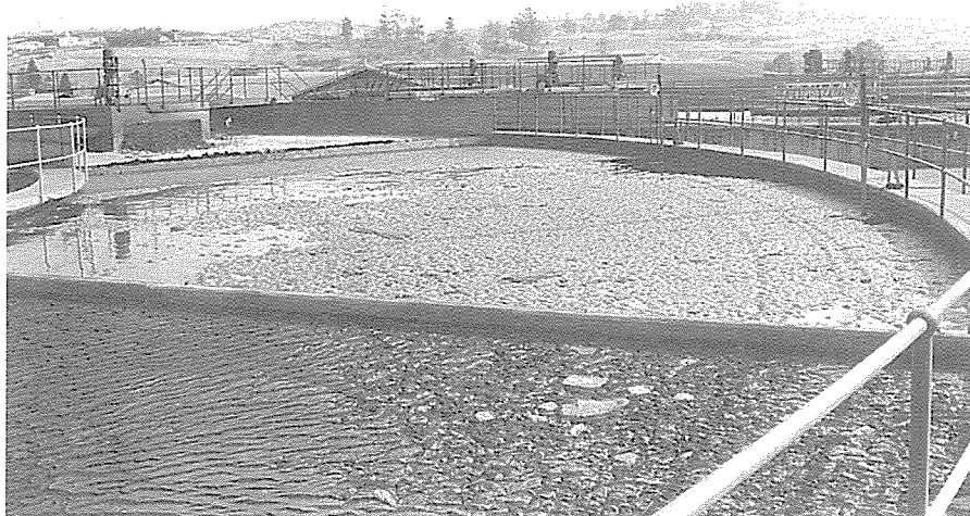
The anaerobic and primary anoxic zones of the Bardenpho reactor.
