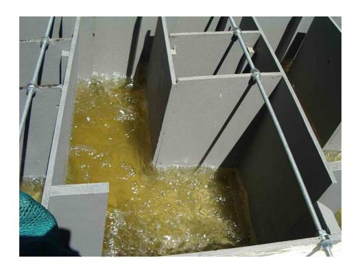
Plate 17: Fishway channel without stones on bottom at ca 8 ℓ/sec discharge
