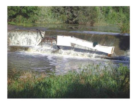
Plate B.2: Fishway set up on the lower shelf at the base of the Kowie weir
