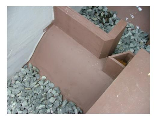
Plate A.3: Sloping sills and substrate incorporated into a modified design.
