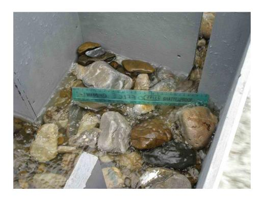
Plate 18: Fishway channel showing stones on bottom at low flows (large fishway channel).
