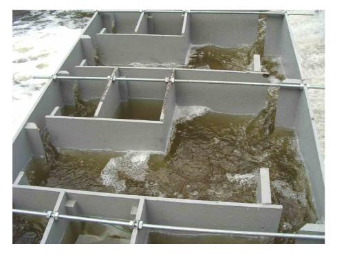
Plate 19: Fishway channel at high flow (18.9 ℓ/sc)
