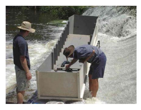
Plate B.1: Setting up the fishway at the Kowie Weir
