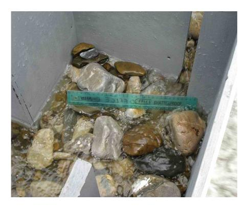
**Plate B.5:** Fishway channel showing stones on bottom at low flows (large fishway channel).
