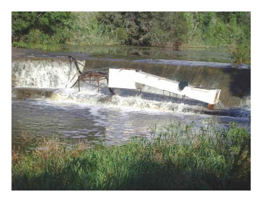
Plate 16: Fishway set up on the lower shelf at the base of the Kowie River weir
