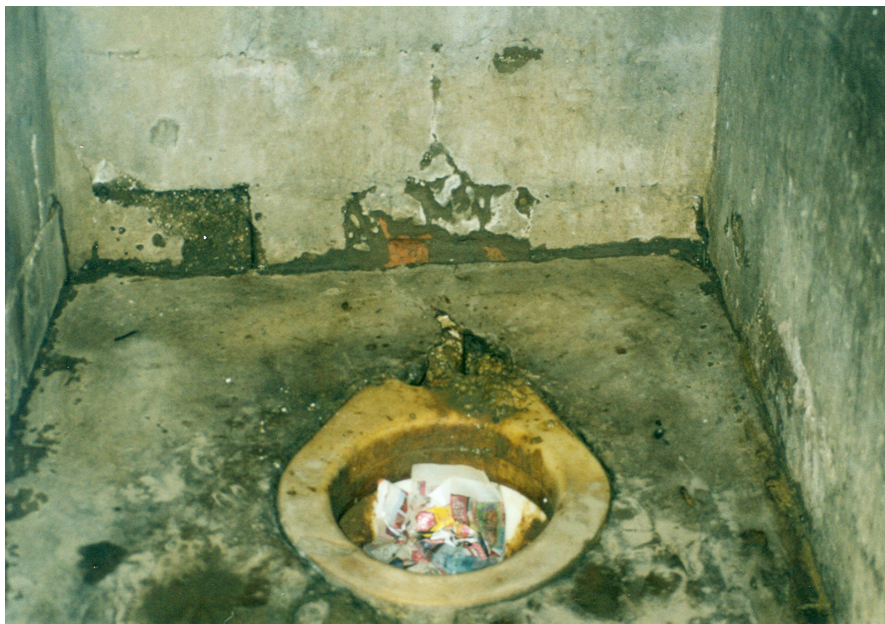
Fig. 2 Toilets blocked, pipes worn out and walls cracked
