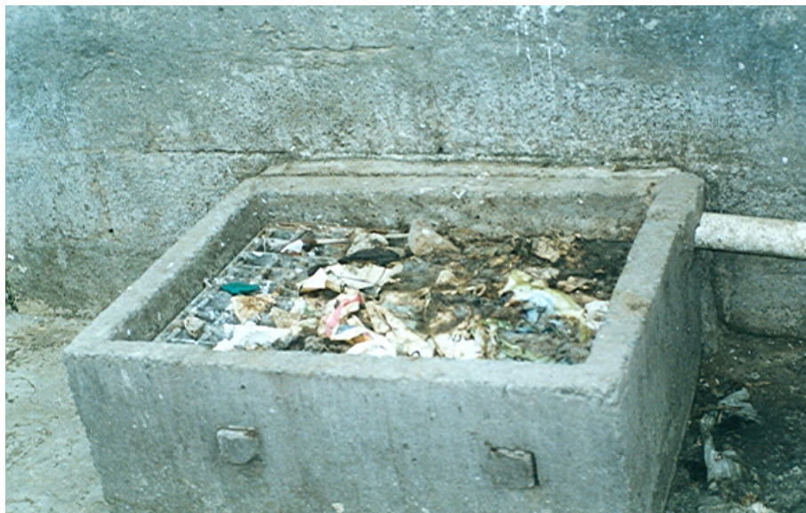
Fig. 4 Drain with plastics and faeces
