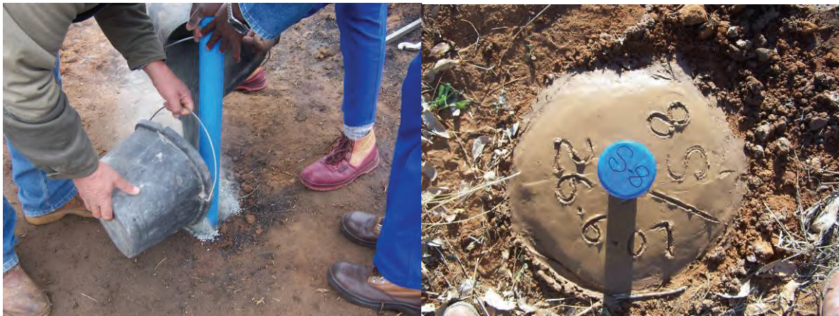
Figure 21: Add filter material and seal the piezometer.
