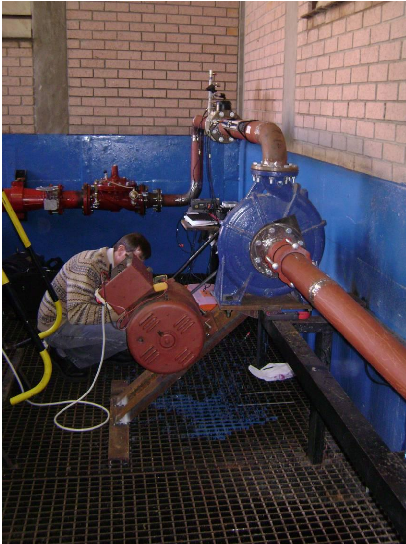
Figure i: Hydropower generation on the inlet side of the Queenswood Reservoir
