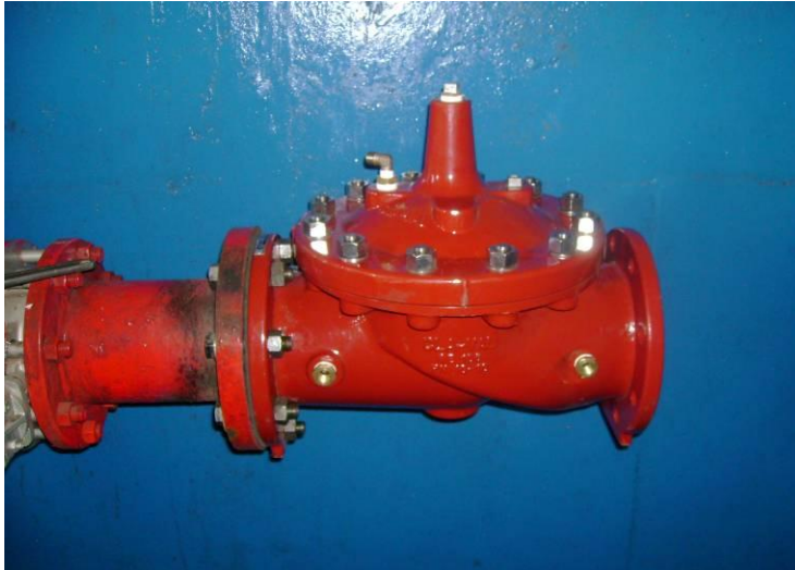
Figure 4.13: Pressure reducing valve installed upstream of pump
