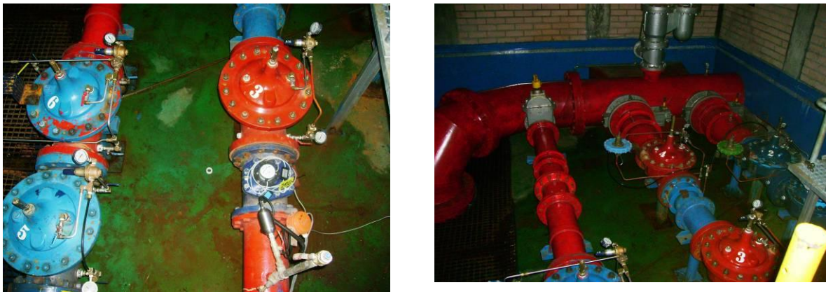
Figure 4.4: Altitude valve configuration in the Queenswood reservoir valve control room
