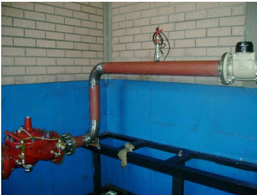
Figure 4.16: Section of bypass before pump-as-turbine
