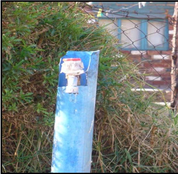
Figure 4.3 Communal standpipe leaking water
