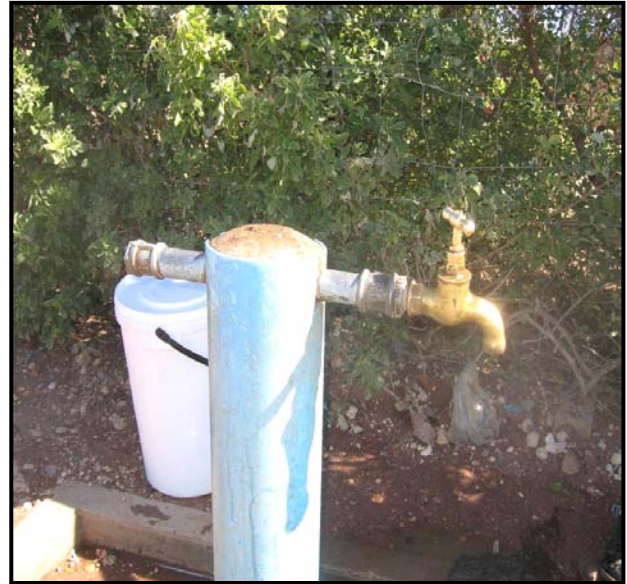
Figure 4.4 Heads broken of the standpipes
