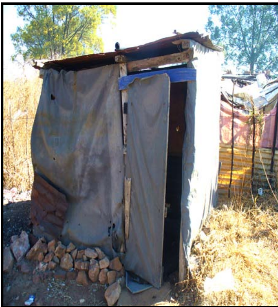
Figure 5.7 Sub-standard toilet structure in peri-urban areas
