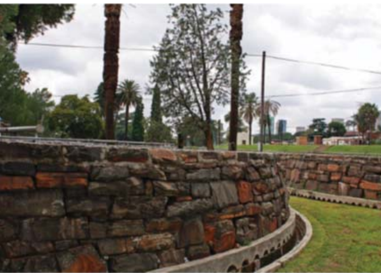
The original biological filtration units are still in use. Image credit: Lani van Vuuren
