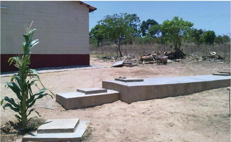
*A typical septic tank and soak pit.*
