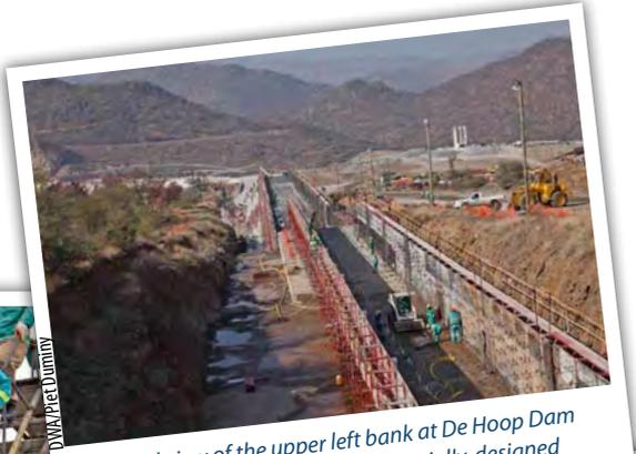
A general view of the upper left bank at De Hoop Dam as it stood in June 2011. Note the specially-designed scaffolding.
