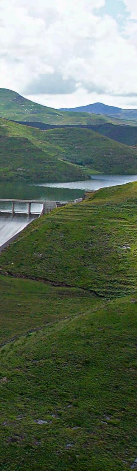
*Left: Mohale Dam is a concrete-faced rockfill embankment, 145 m high. Here the ungated spillway, built on the left abutment of the dam, can clearly be seen.*
