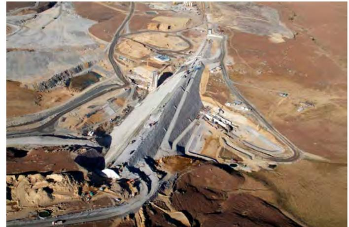
downstream side of this pre-cofferdam the main cofferdam was then constructed to commence with the peat excavation.
