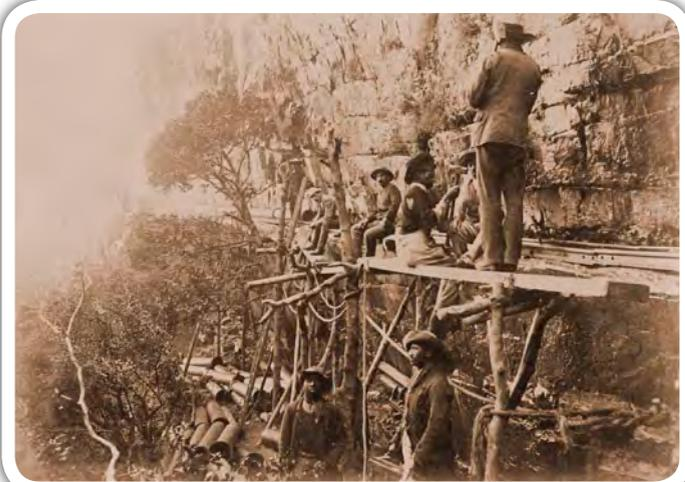
*Left: Labourers working on the Woodhead Dam wall. Note the primitive wooden scaffolding.*
