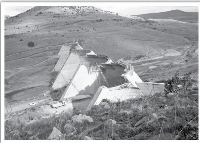
**Top right:** Wagendrift Dam nearing completion. Some of the shuttering can still be seen. The dam used the same type of shuttering as that applied on the construction of Kariba Dam.
