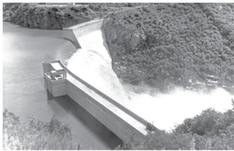
**Right:** A close-up view of the Blyderivierspoort Dam overspill section. The steps built in to dissipate the energy of the falling water can clearly be seen.
