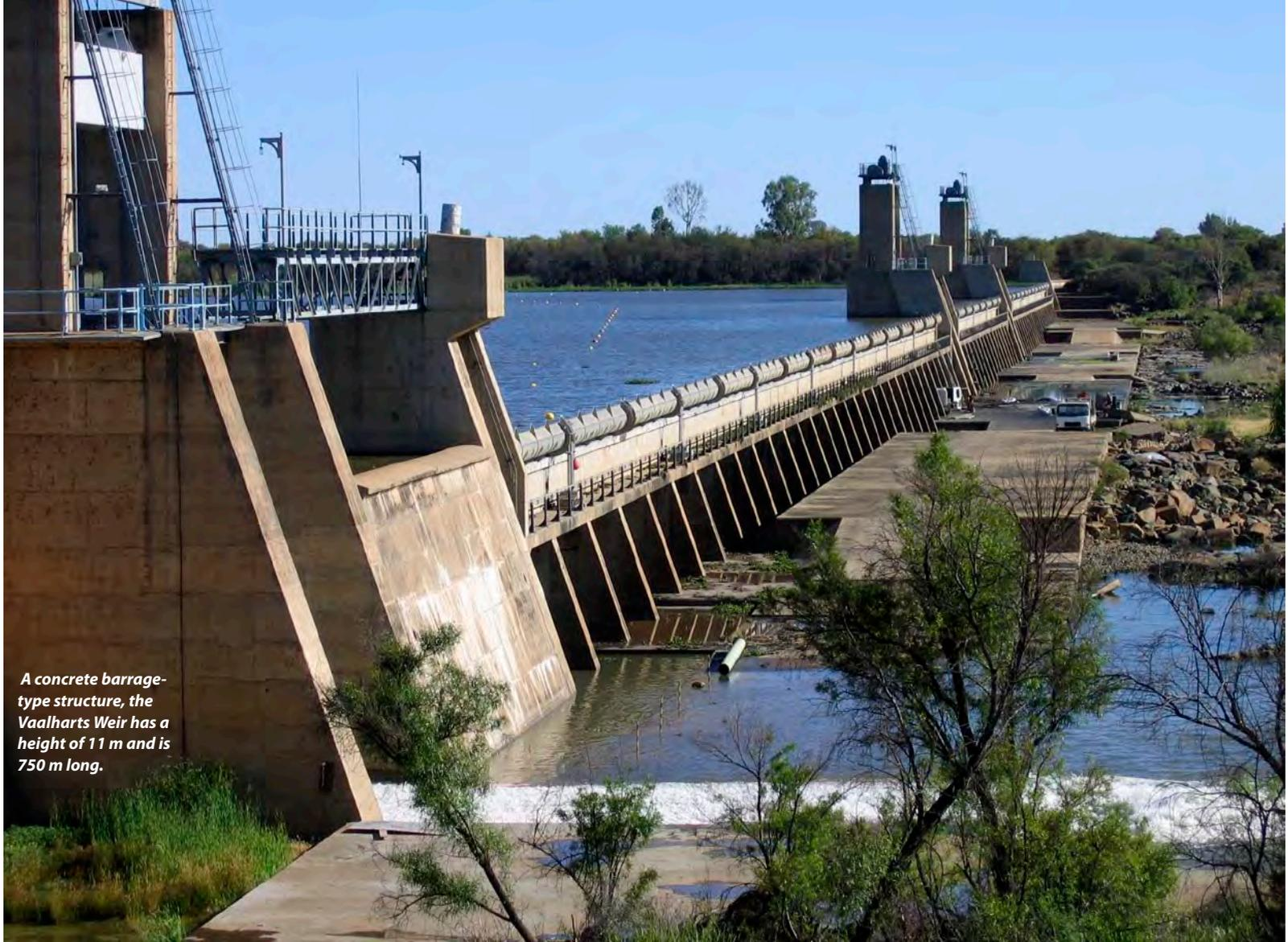
*A concrete barrage-type structure, the Vaalharts Weir has a height of 11 m and is 750 m long.*
