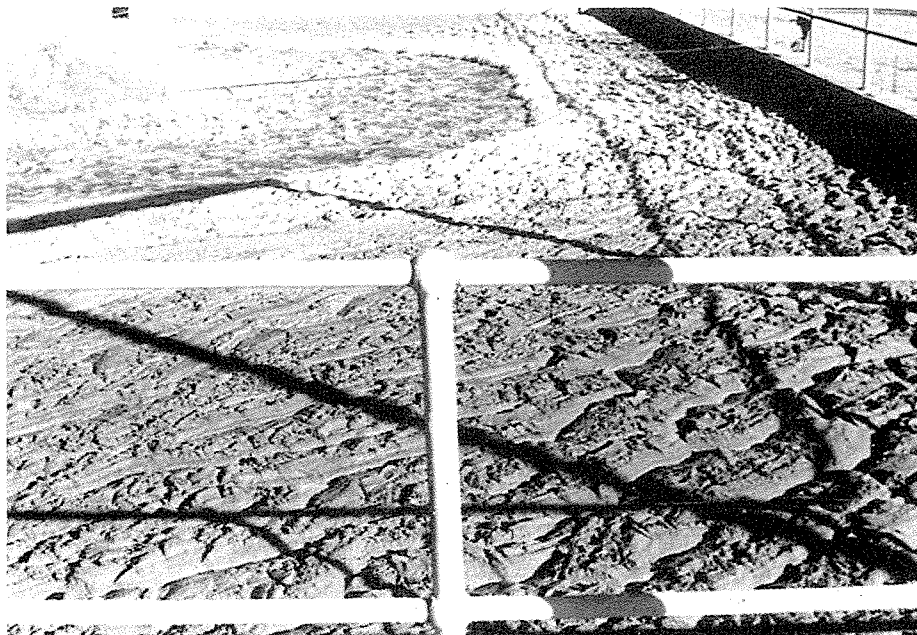
Biological foaming at the Randfontein Estate Gold Mine activated sludge plant. M. parvicella are the dominant foam bacteria.
