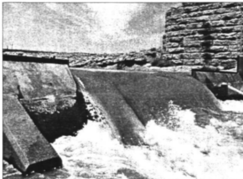
Figure 1.1: Compound sharp-crested weir
