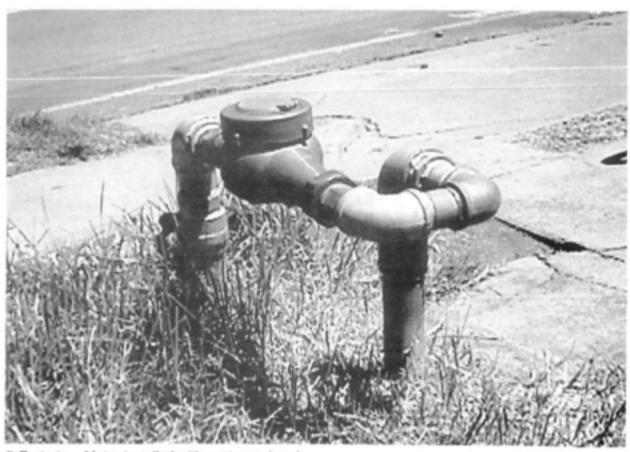
f) Pretoria - Meter installed with upstream bends
