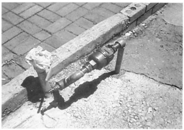
e) Pretoria - Meter installed in a skew pipe arrangement
