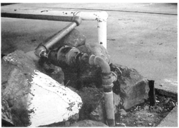
c) Pretoria - Meter installed with upstream bends
