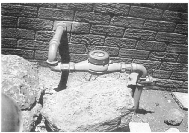
a) Pretoria - Meter installed with upstream bends
