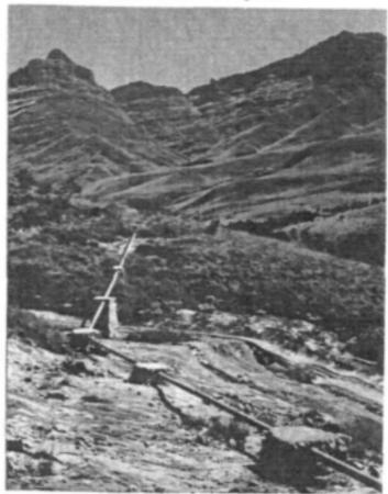
Bulk supply pipeline from weir, Tsita Project
