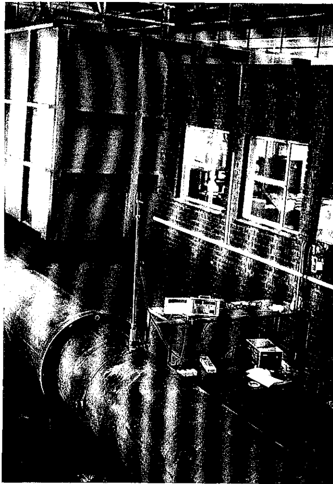
Insertion Meter installed on 800 mm dia pipeline. Weigh tank and control room in the background.
